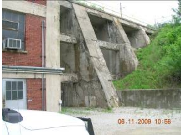
Figure A5-1: Depiction of failure mode and example of freeze-thaw in a buttress dam, Bureau of Reclamation.
