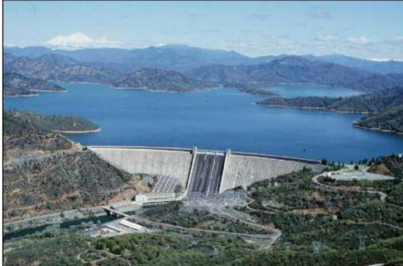
Figure A1-4: A curved gravity dam, Bureau of Reclamation.
