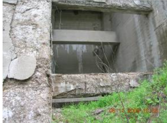
Figure A5-1: Depiction of failure mode and example of freeze-thaw in a buttress dam, Bureau of Reclamation.
