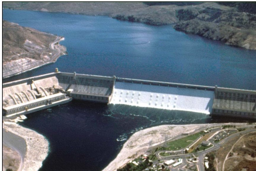
Figure 2-1: Gravity dam, Bureau of Reclamation.
