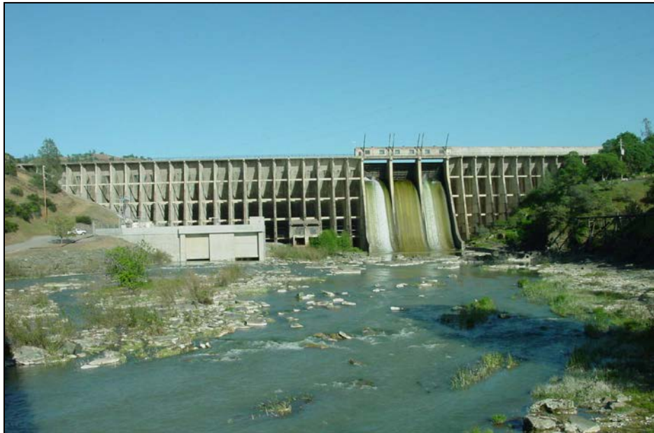
Figure A4-1: Downstream side of a slab and buttress dam, Bureau of Reclamation.
