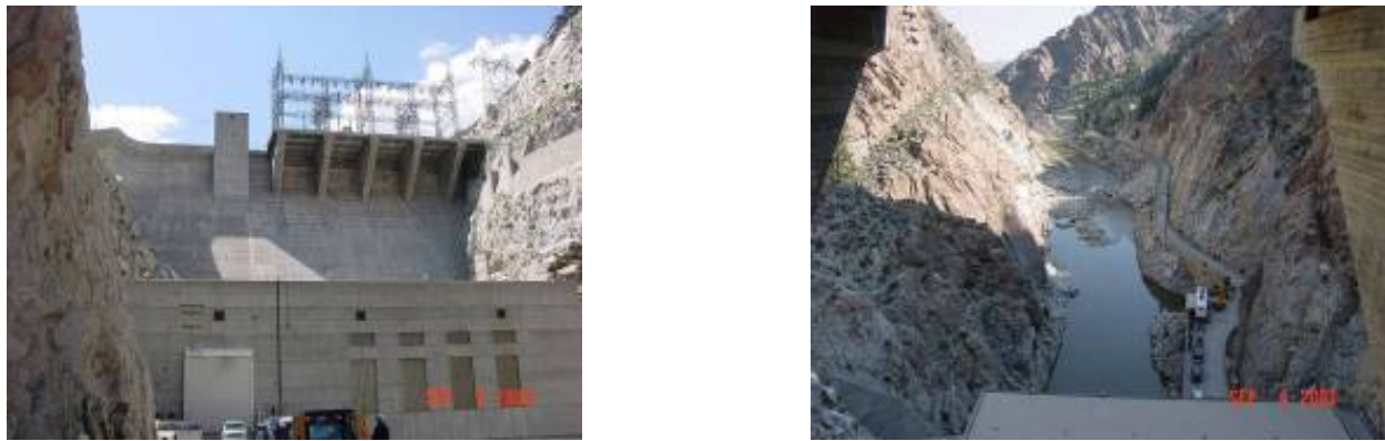
Figure A1-5: Looking upstream and downstream from a gravity dam in a narrow canyon, Bureau of Reclamation.
