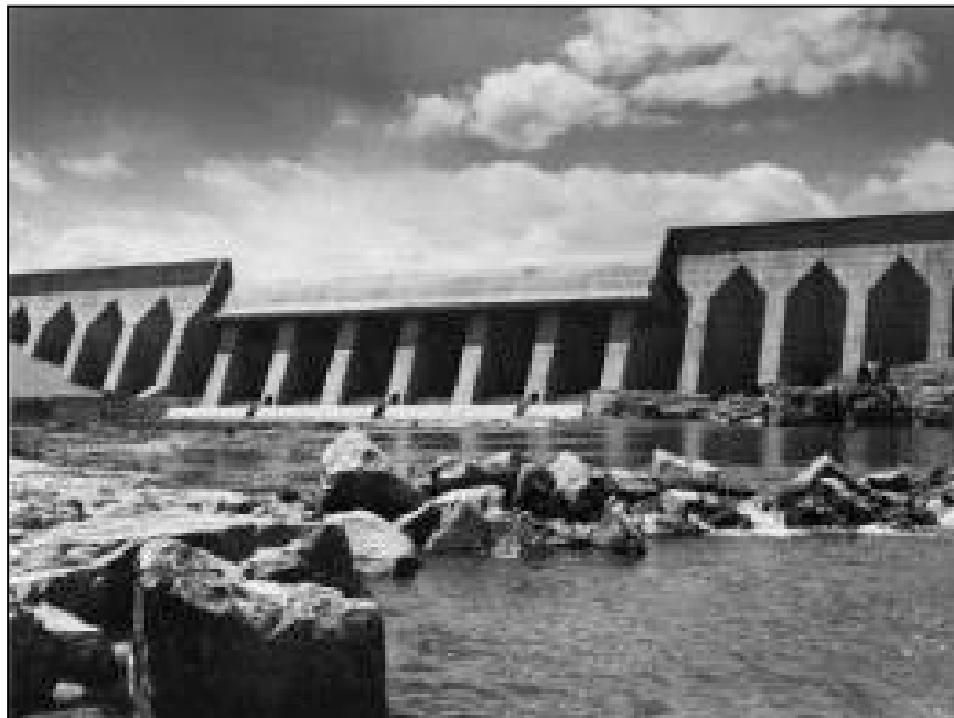
Figure 2-4: Massive-head buttress dam, Bureau of Reclamation.
