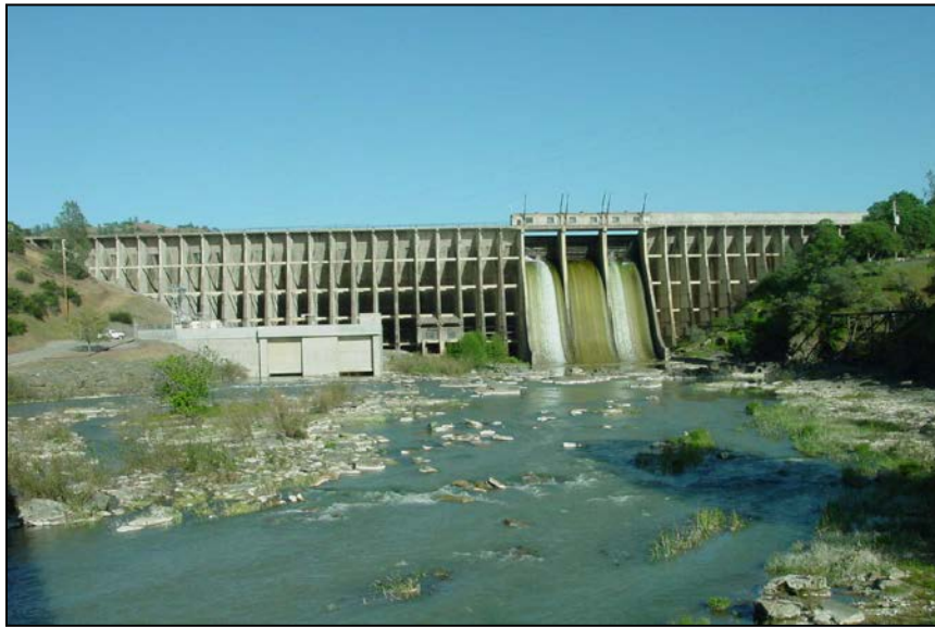
Figure 2-3: Slab and buttress dam, Bureau of Reclamation.
