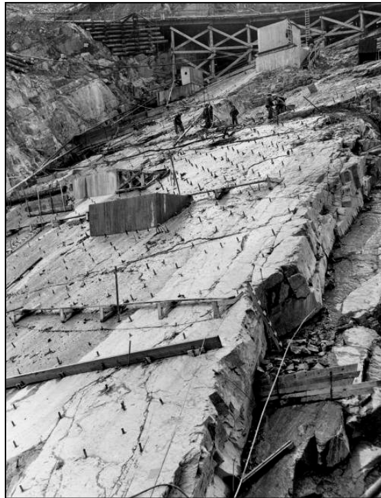
Figure A3-5: This photograph, taken during construction, shows dam-to-foundation contact and the continuous nature of slide planes on the left abutment; the side plane is the fault just below workers, the base plane is parallel to dam contact, and the release plane is vertical along the upstream face of the dam, Bureau of Reclamation.
