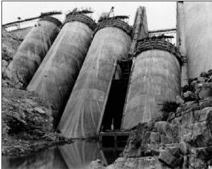
Figure 2-5: Multiple-arch buttress dam, Bureau of Reclamation.
