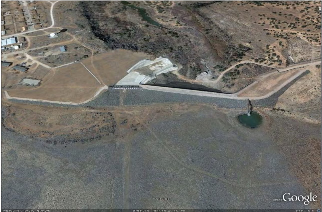
Figure 6.—Oblique view of modified Black Rock Dam (Google Earth, October 30, 2012).
