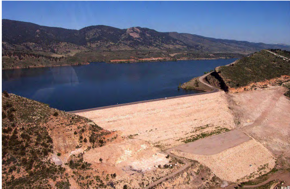
Figure 10.—Completed downstream modification at Dixon Canyon Dam.
