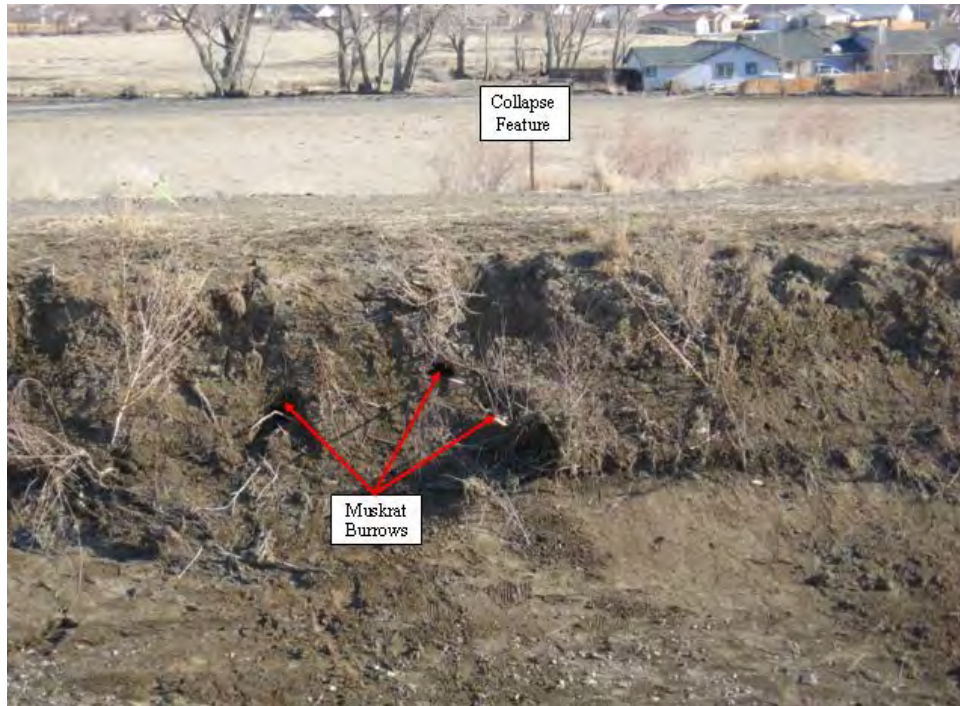
Figure 11.—View of canal embankment prior to investigations showing three muskrat burrow entrances on the waterside and the location of a collapse feature (feature not visible) on the landside. The burrow entrance appeared to be located a foot or so below the approximate 350 ft 3 /s flow line.
