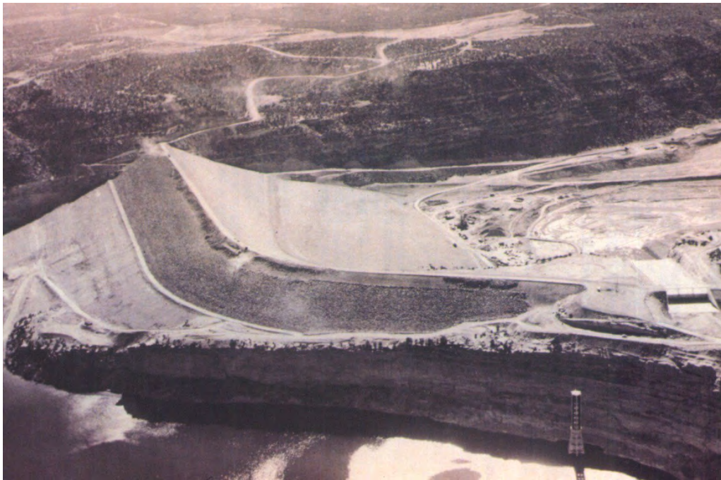
Figure 2.—Right abutment of Navajo Dam, looking downstream.
