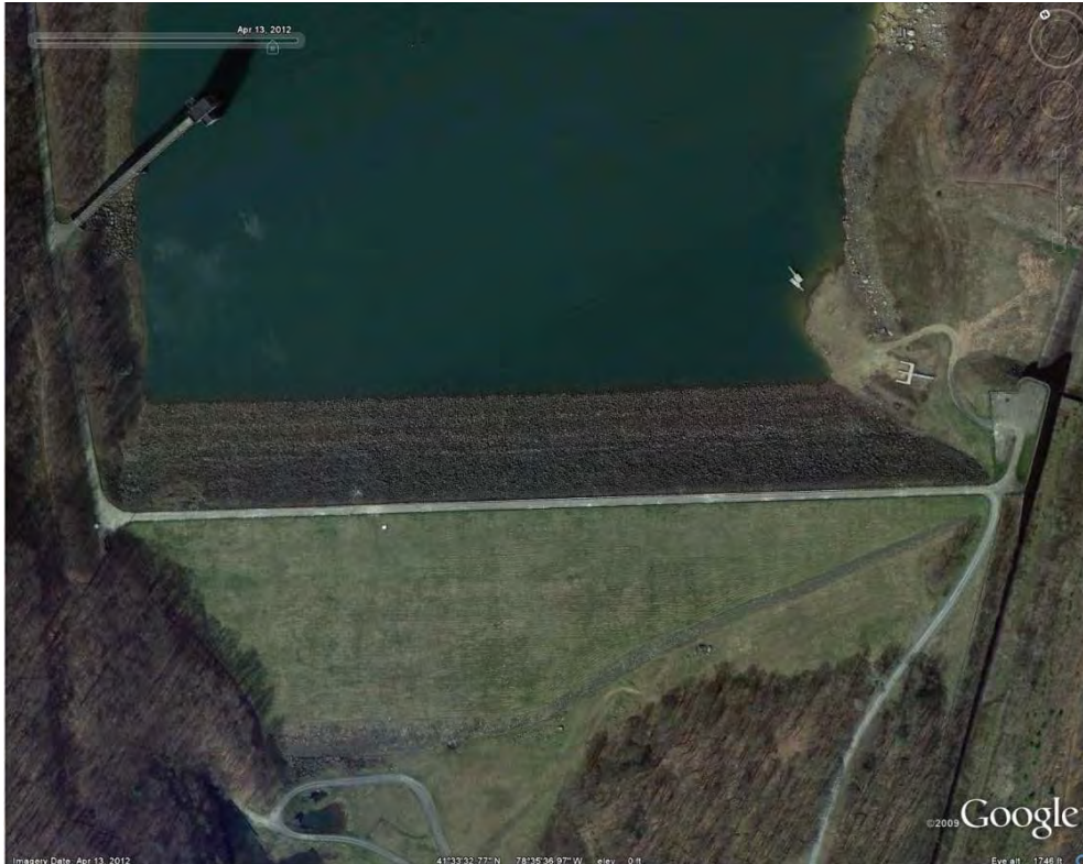
Figure 1.—East Branch Dam – the incident occurred over the steep, right abutment (Google Earth, April 13, 2012).
