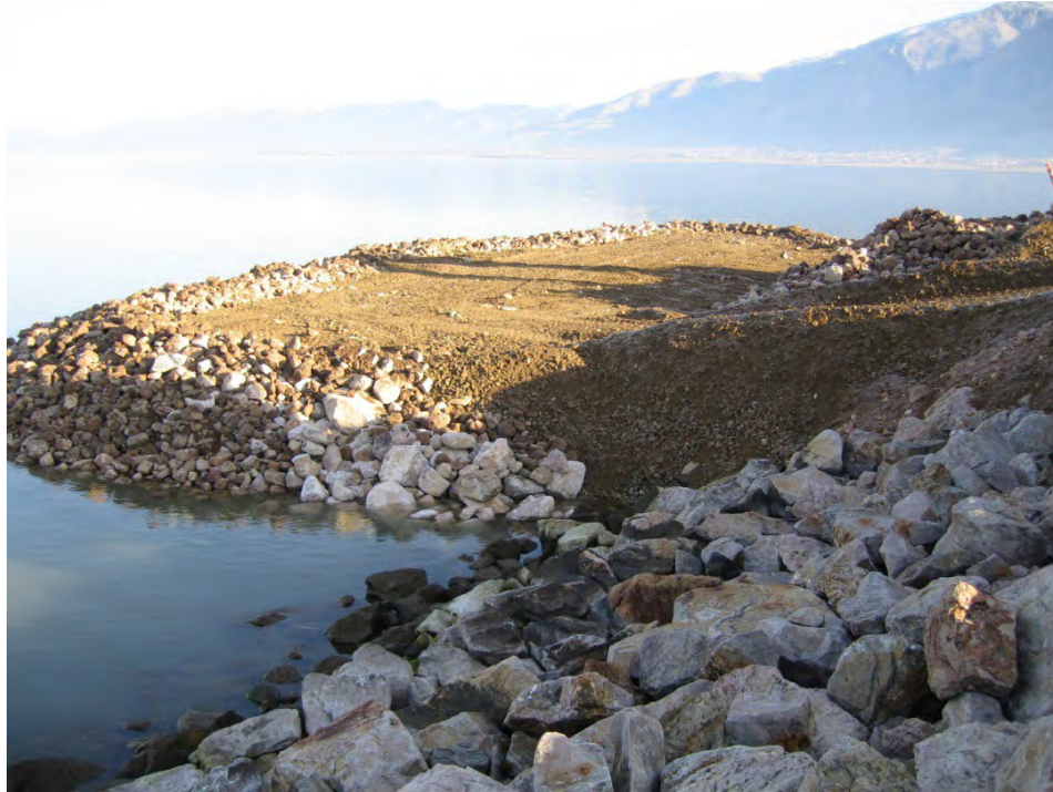
Figure 5.—Erosion into the South Drain did not stop until an upstream berm of gravel and pit-run material was pushed into reservoir.
