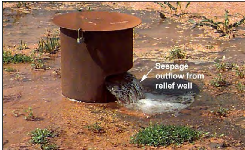
Figure 7-9.—Relief well seepage outflow. Although relief wells are not typically installed for the primary purpose of seepage water monitoring, their outflow can be collected, measured, and evaluated similar to open piezometers or observation wells.
