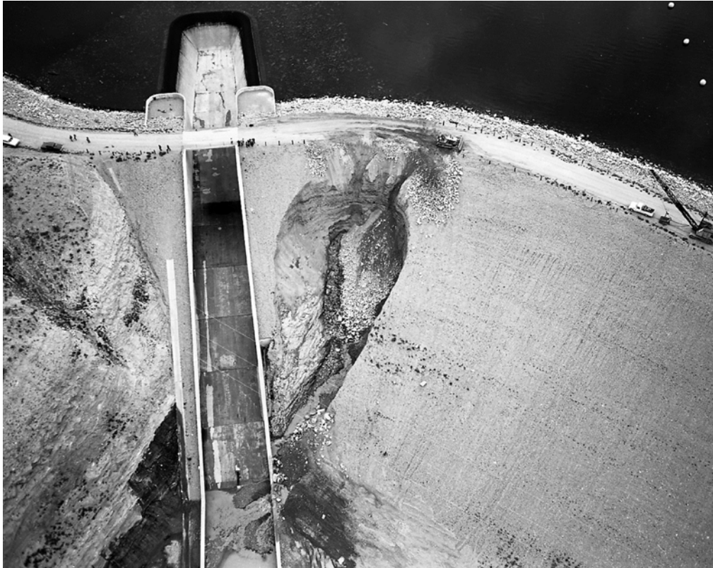
Figure 4b.—The sinkhole migrated in the upstream direction, expanding in size, as material progressively caved from the sides and was washed out of the bottom (stopping).
