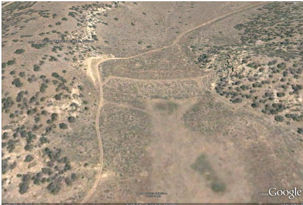
Figure 1.—Oblique view of Cañon C-4 Dam, looking downstream (Google Earth, June 22, 2005).
