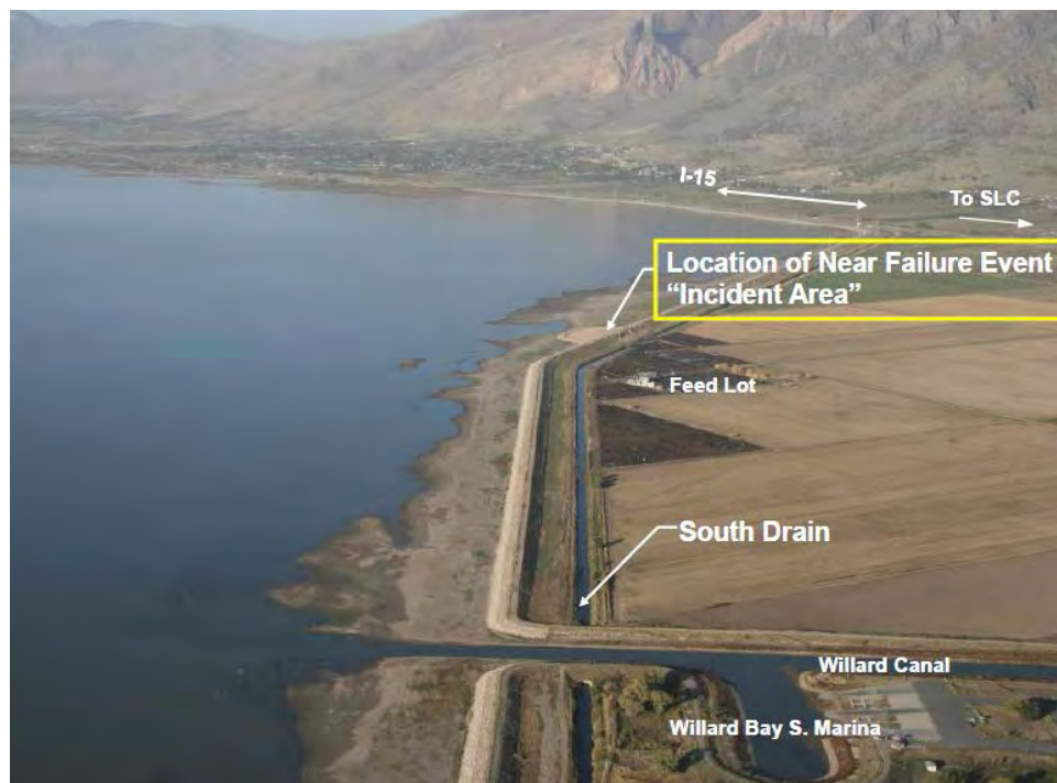
Figure 4.—Aerial view of the western portion of the dam showing the incident location in relation to the South Drain and feedlot.
