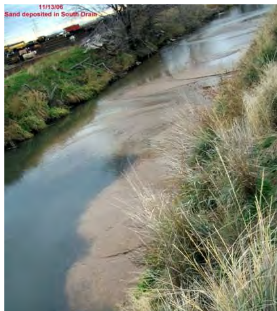
Figure 6-1.—Visual observation of failure mode in progress.
