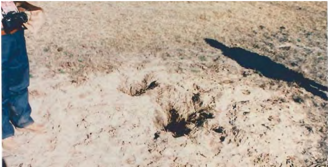
Figure 6.—Tunnel outlet downstream from Sta. 5+50, March 8, 1988.
