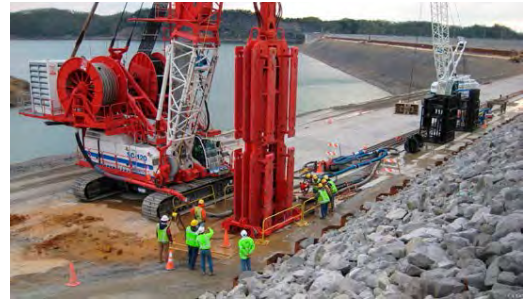
Figure 9.—View of hydromill construction.
