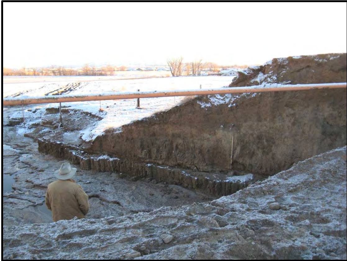
Figure 3.—View through the breach toward Fernley, Nevada. The downstream breach face cut into the left canal embankment is 17½ ft high.
