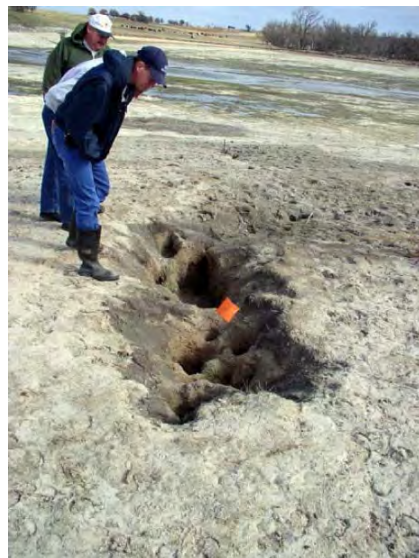
Figure 10.—Large sinkhole in reservoir.
