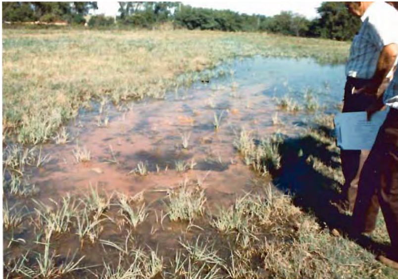
Figure 5.—Seepage occurring downstream from embankment in September 1987.
