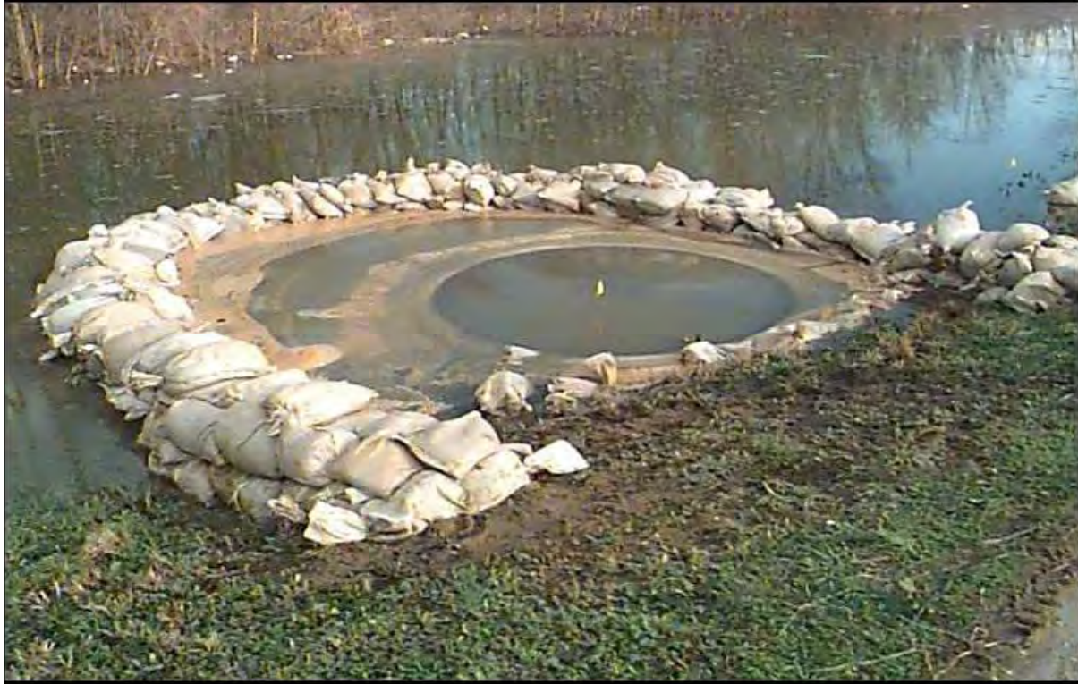
Figure 10-14.—Sandbags placed around a sand boil to increase tailwater level as part of a temporary risk reduction measure. (Photo courtesy of USACE, Missouri Valley Division)
