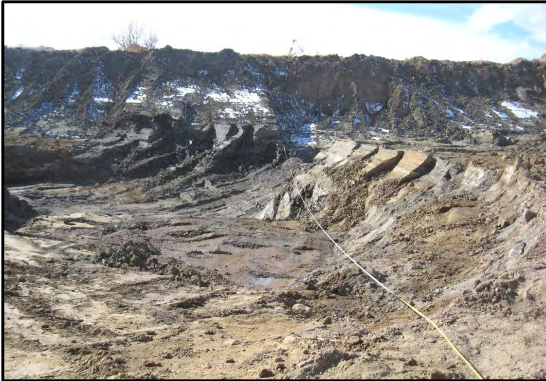
Figure 8.—View to the southwest (toward the right side canal embankment) of the final excavation of the scour hole site.
