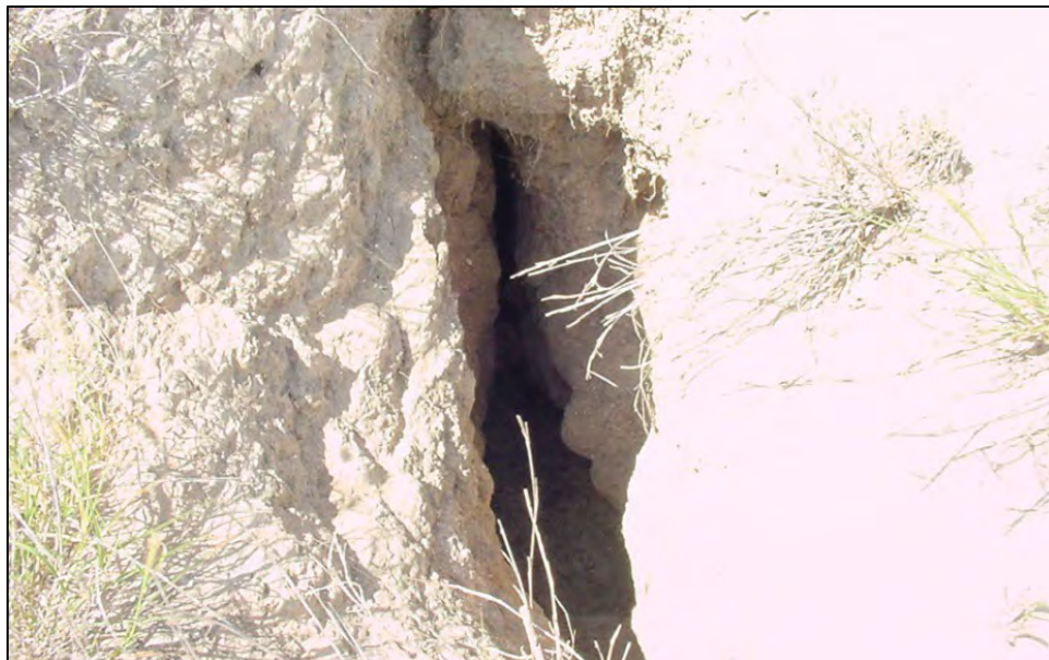
Figure 2.—Large crack in embankment, Olmitos-Garcias No. 2 Dam.
