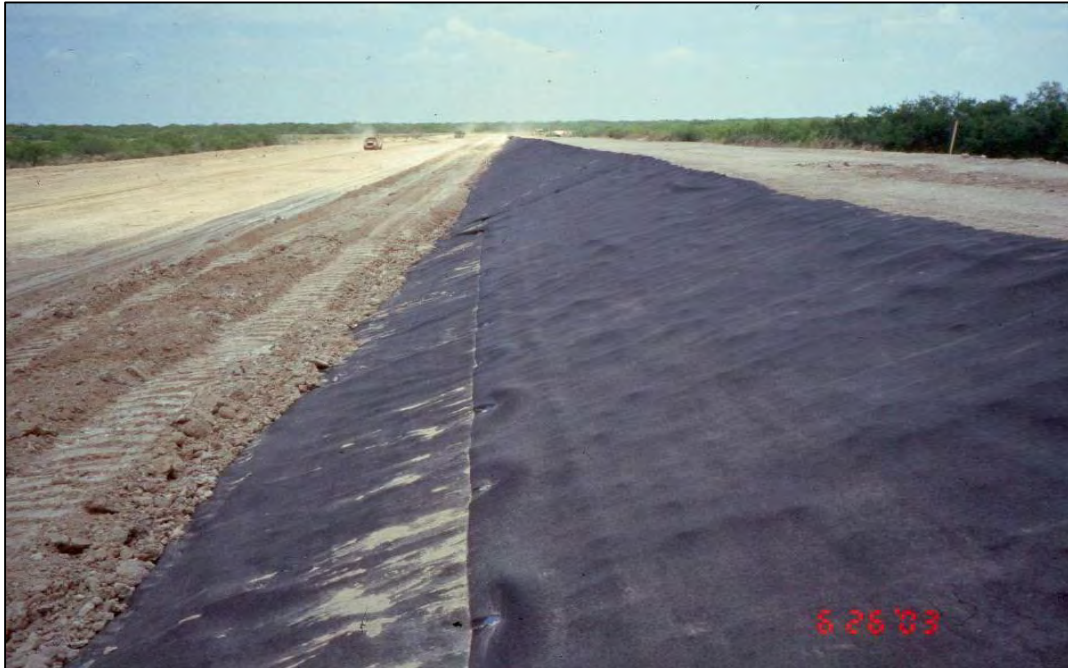
Figure 6.—Fill placement against geotextile, Olmitos-Garcias No. 2 Dam.
