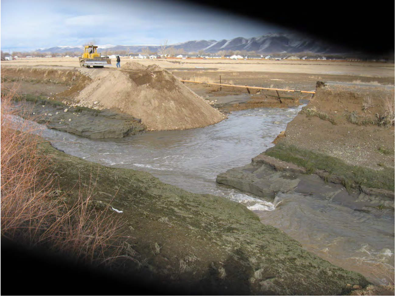
Figure 1.—Photo of the breach during early phases of temporary breach repair on the morning of January 5, 2008. Normal canal flow is from left to right in this photo. The breach is being filled by pushing fine-grained soil into the gap in the canal embankment. Some of the scour of the canal bottom can be seen along with some scour of the area immediately downstream from the breach. The pipeline shown is an abandoned natural gas pipeline that had been buried in the canal embankment. The pipe remained in place after the breach despite eroding all support provided by the original embankment.
