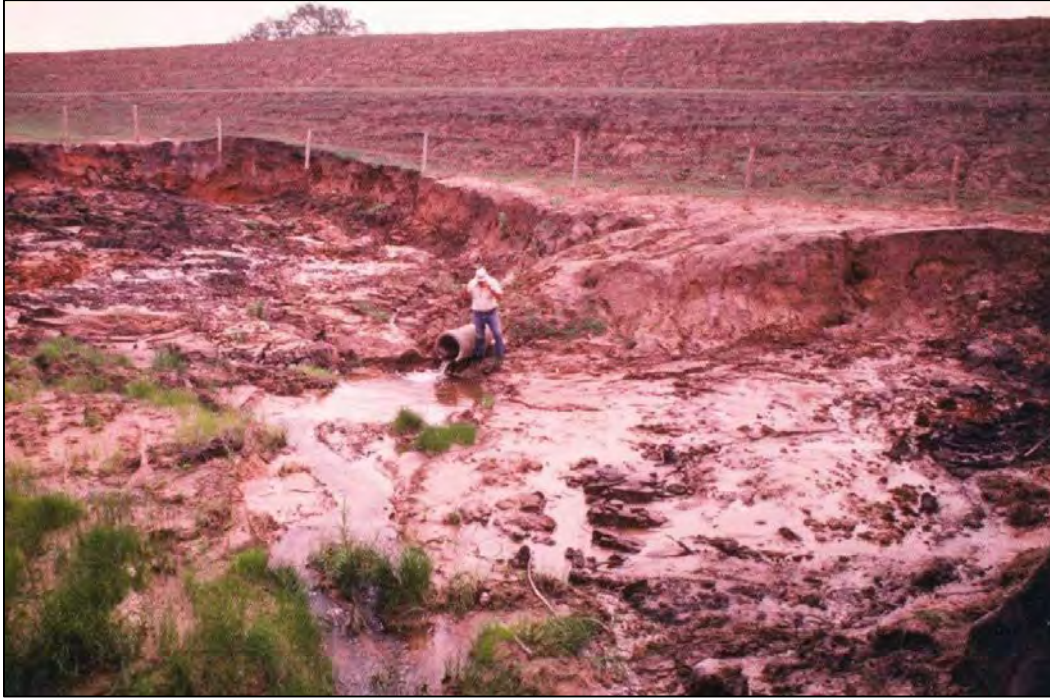
Figure 10-21.—Seepage-caused slope instability near outlet of principal spillway conduit, Little Washita No. 13, Oklahoma (1979). (Photo courtesy of NRCS, Oklahoma)
