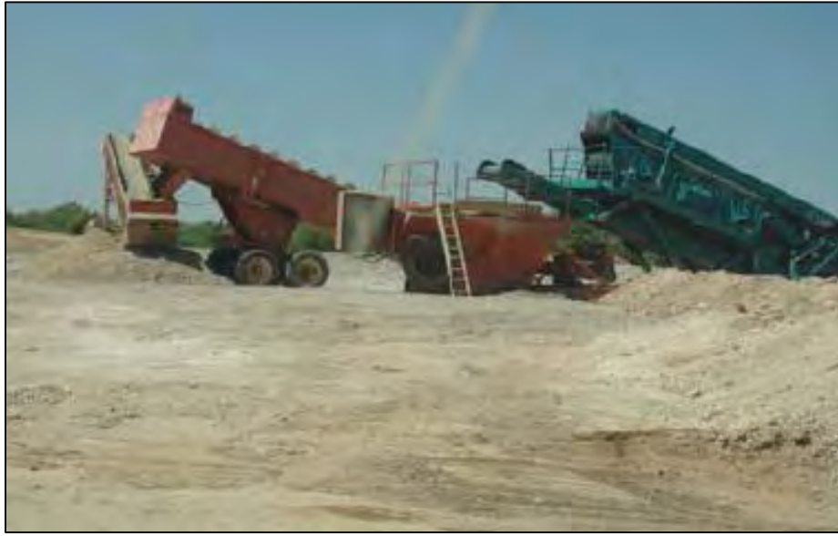
Figure 4.—Screening machine (right) and mixer/elevator (left) for processing filter material, Florence Dam.
