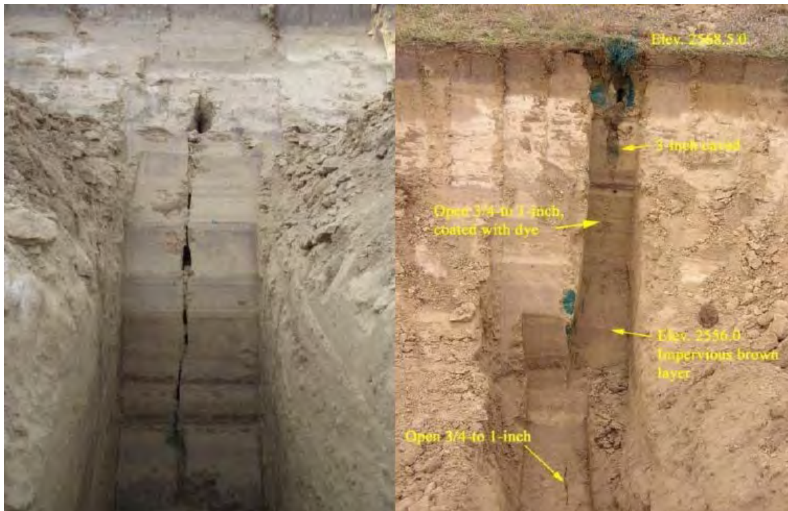
Figure 5.—Representative cracking in the embankment observed in test pit #2. Dye was poured into the sinkholes to aid in tracing the cracks. Cracks were typically 1/4 to 1 in wide.
