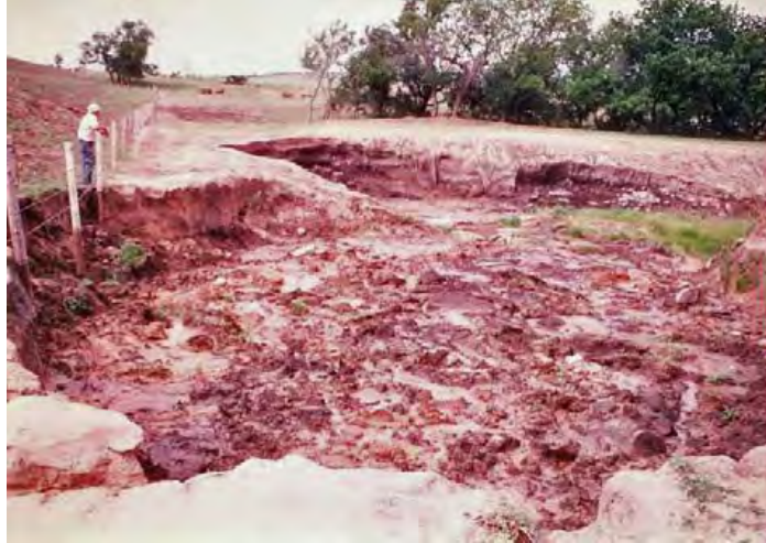
Figure 4.—Sloughing of downstream area observed in May 1979.
