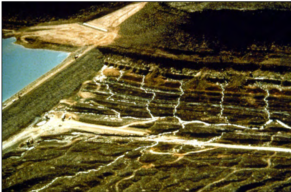
Figure 5.—Excessive leakage during first filling.
