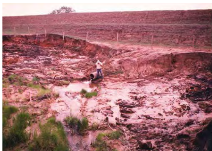
Figure 3.—Sloughing of downstream area near plunge pool.
