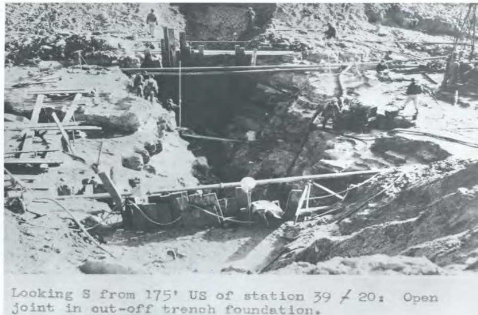
Figure 3.—Solutioned dolomite observed in cutoff trench.
