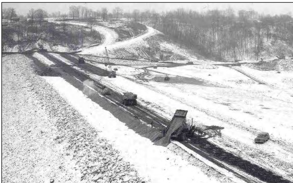
Figure 3-4.—Examples of winter construction at embankment dams prior to removal of snow and ice contamination. (Top) Blue blanket is insulated to prevent freezing of underlying soils. (Bottom) Placement of fill on improperly prepared frozen ground, snow, and ice.
