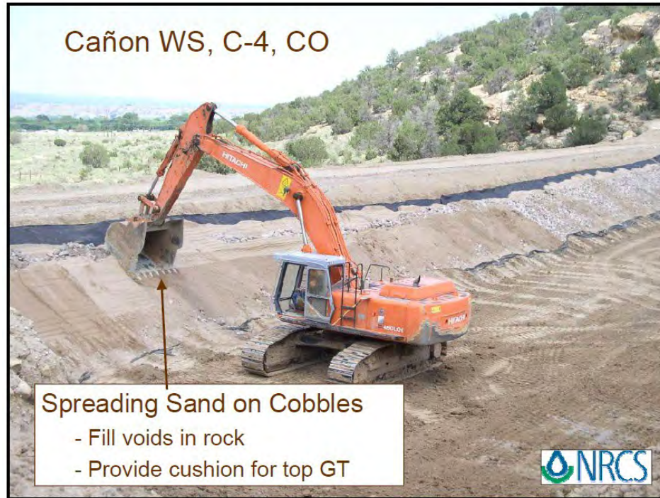
Figure 8.—Placement of geotextile, rockfill, and sand on upstream face (prior to placement of overlying geotextile).
