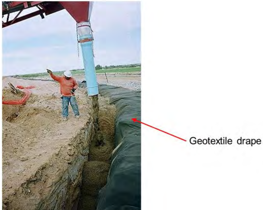
Figure 5.—Placing filter material with tremie, Florence Dam.
