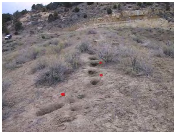
Figure 2.—Holes observed in crest.
