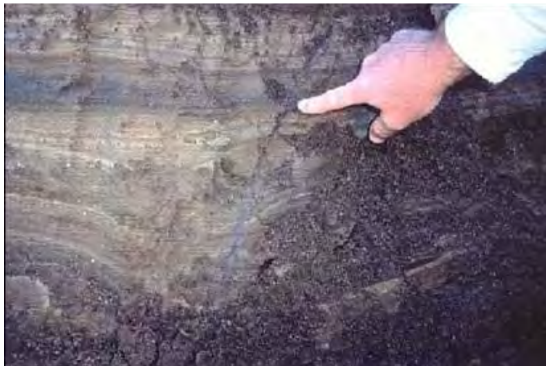
Figure 3-3.—Suspected hydraulic fracture at Ochoco Dam near the intake tower that was subsequently filled with reservoir sediments.
