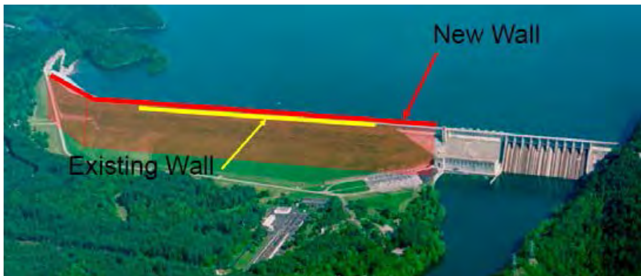
Figure 2.—Overall view of the dam showing extent of the existing and new cutoff walls.
