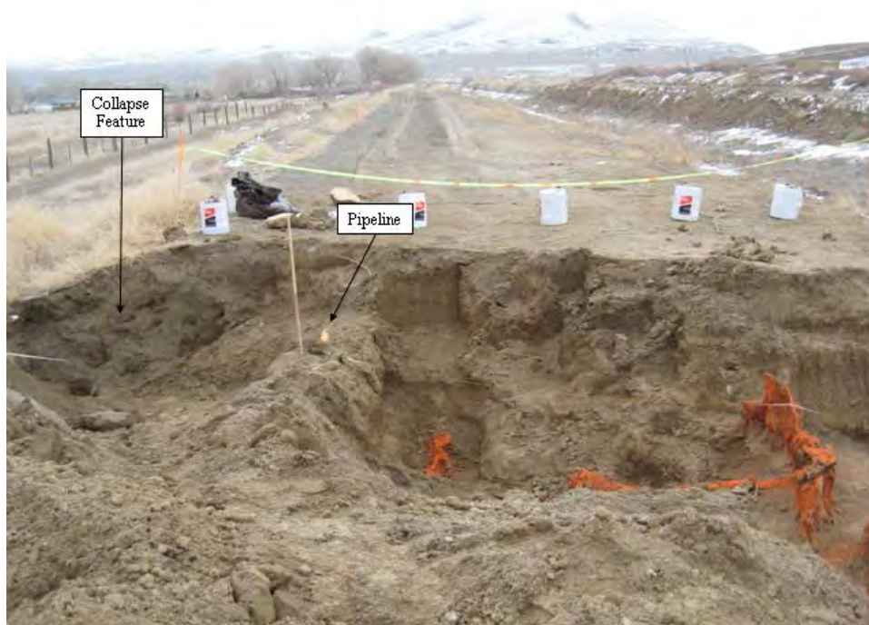
Figure 10.—View of partial excavations of canal embankment crest following grouting with Stratathane™. Features that were found grouted have been painted with orange paint.
