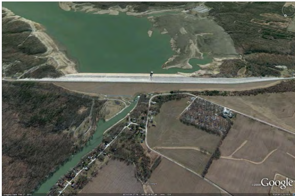
Figure 2.—Oblique view of dam (Google Earth, February 27, 2012).
