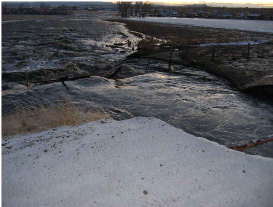
Figure 5.—Earliest photos showing breach (estimated time about 6:30 a.m. on January 5, 2008) (photos by Walt Winder, TCID).
