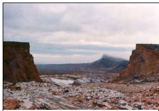
Figure 1b.—Breach through Quail Creek Dike.
