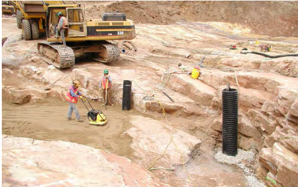
Figure 8.—Foundation cleanup and construction of downstream filter and berm at Spring Canyon Dam.
