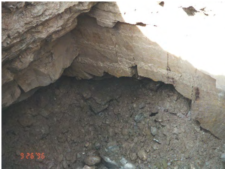
Figure 4.—Looking into sinkhole from foundation contact.
