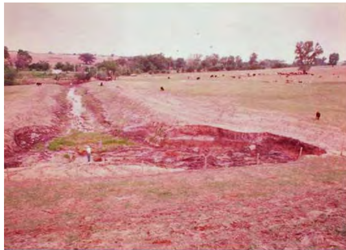
Figure 2.—Sloughing of plunge pool in May 1979.
