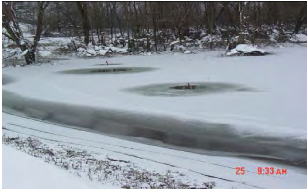
Figure 6-11.—Seepage water discharge locations (flagged with red markers) are more evident during the winter due to water temperature differences.
