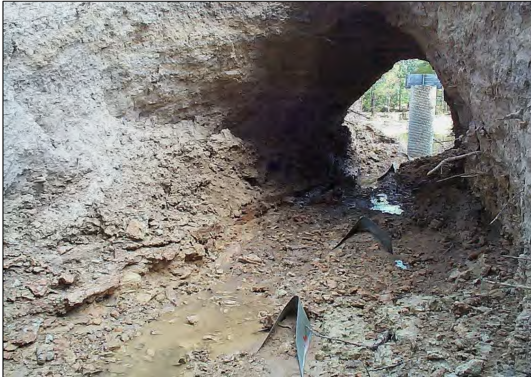
Figure 10-8.—Failure of an earth embankment in Louisiana along the principal spillway conduit, looking upstream toward riser. Notice damaged anti-seep collars on conduit. (Photo courtesy of NRCS, Louisiana)
