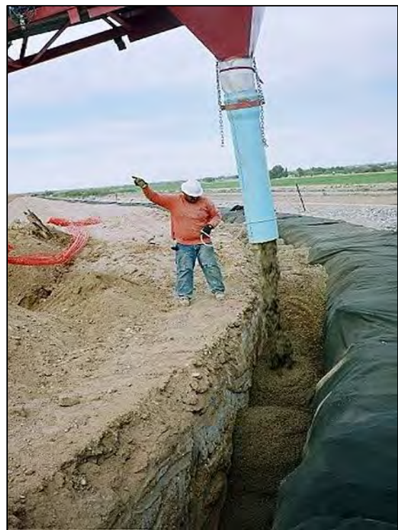
Figure 10-19.—Construction of a geotextile/aggregate chimney filter in Florence Dam in Arizona. Geotextile drape is on right (downstream) side of trench. (Photo courtesy of NRCS, Arizona)
