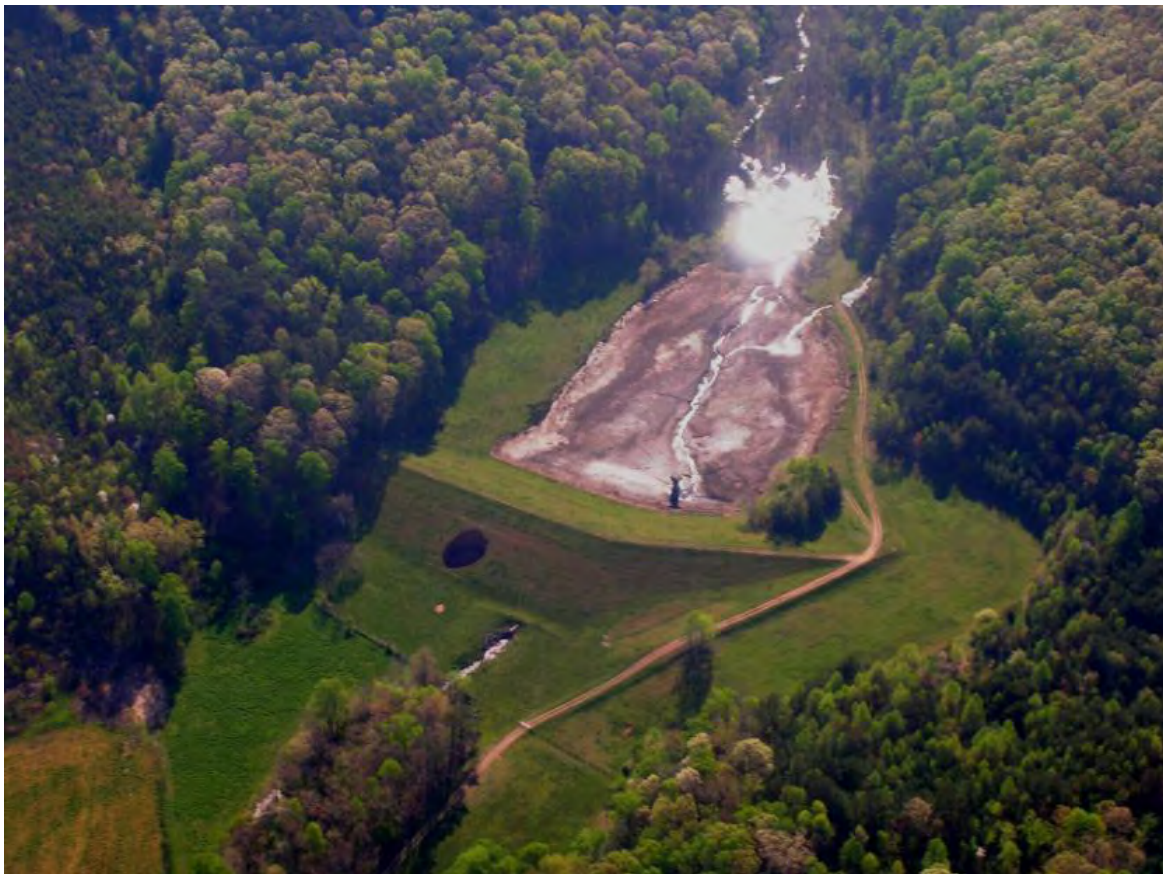
Figure 2.—Aerial view of the sinkhole on the downstream slope of the dam. Photo was taken after the reservoir had been drained.
