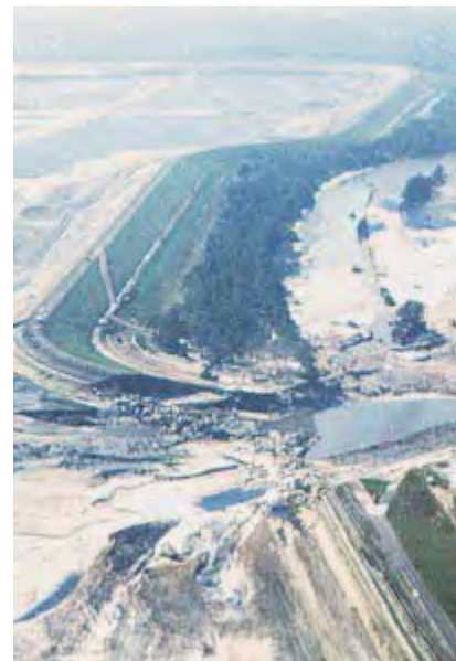
Figure 5.—Same area after breach.
