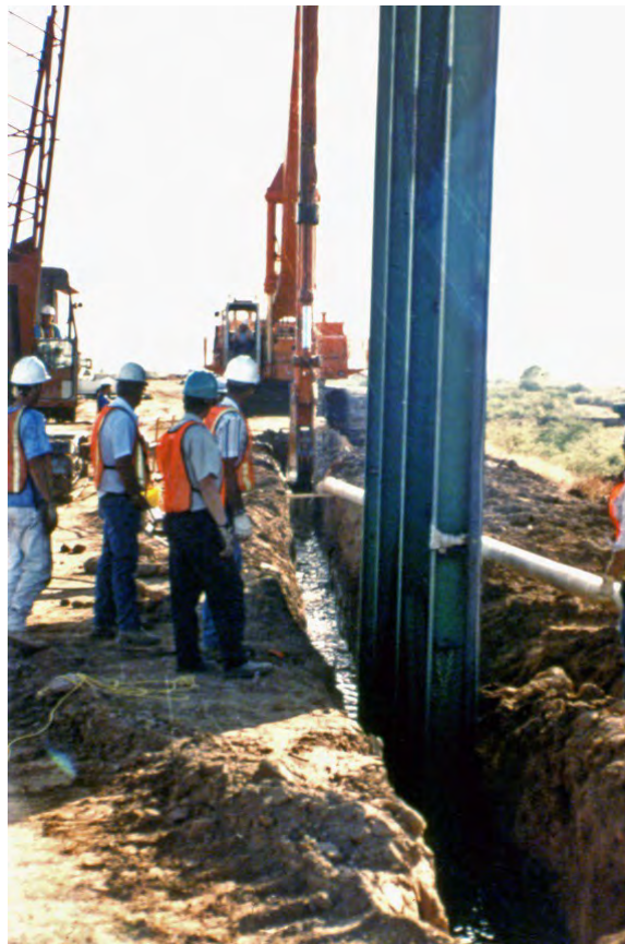
Figure 7.—Excavation of trench using biopolymer slurry. Steel frame was used to install the geomembrane panels.
