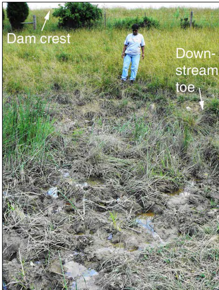
Figure 6-2.—Seepage discharge where the typical grass growth has been retarded in the saturated soil environment and where other vegetation species are becoming dominant.
