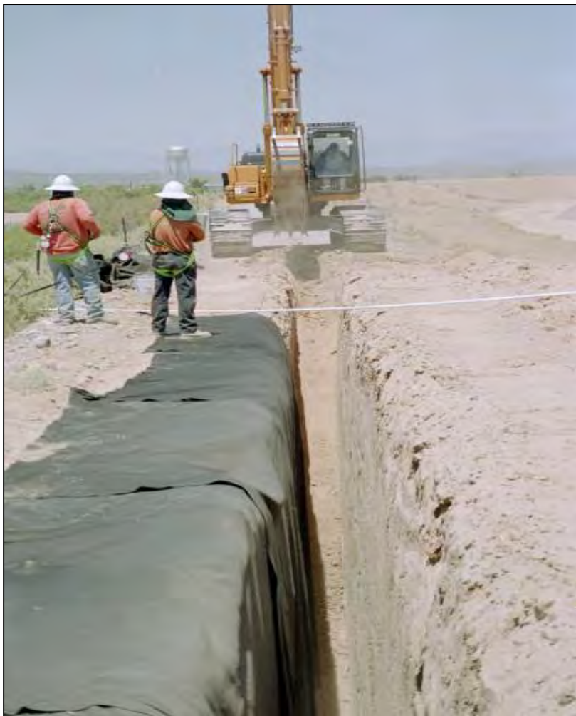
Figure 3.—Trenching and operation, Florence Dam.
