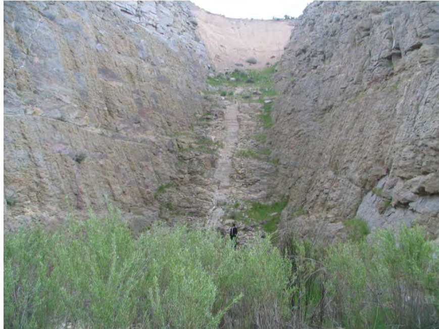
Figure 4.—Narrow, 70-ft-deep abutment cutoff trench. Man shown for scale (photo courtesy of James Wright 2007).
