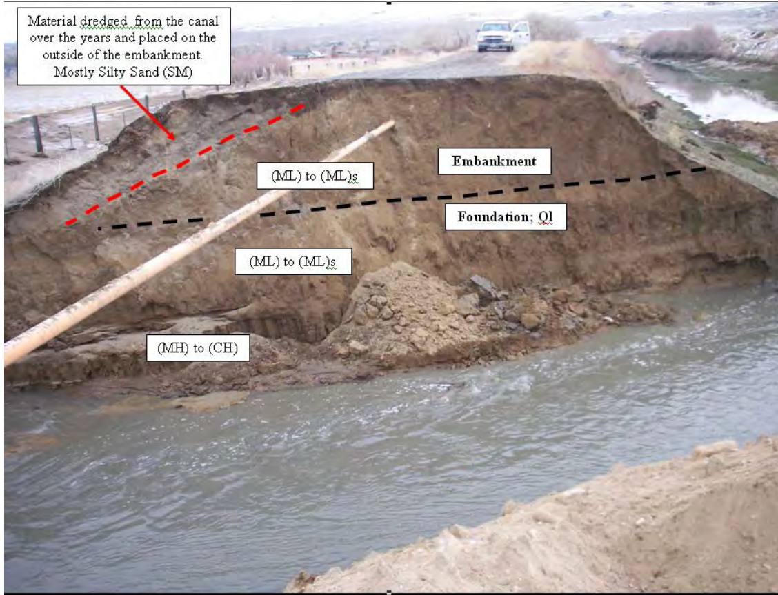
Figure 7.—Downstream view of the Truckee Canal breach. Dashed, black line is the approximate contact between the canal embankment and in-place lakebed deposits (Q1) composed primarily of silt with sand (ML)s and elastic silt (ML) with minor sandy lenses. Center-left is an abandoned Sierra Pacific Power gas pipeline.
