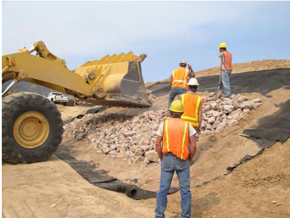
Figure 7.—Constructing the mockup.
