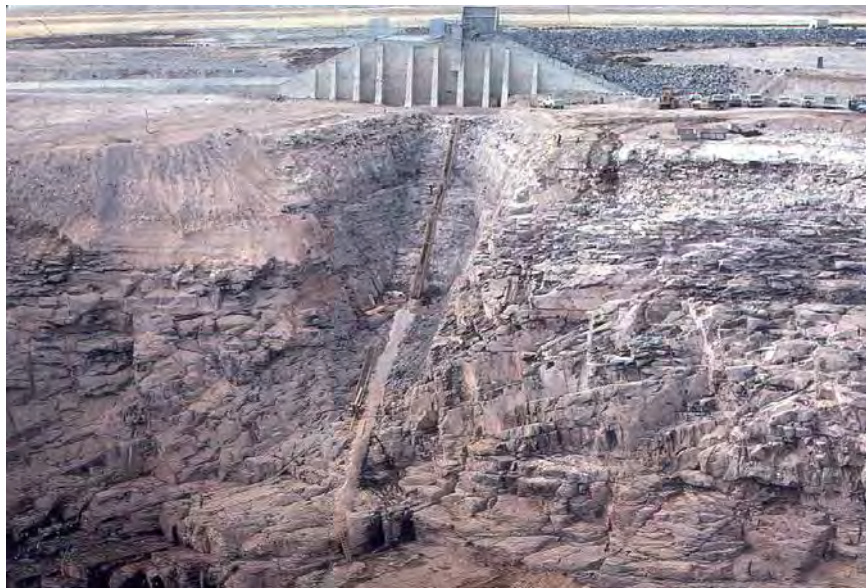
Figure 5.—Deep, highly fracture zone under the right abutment cutoff trench. Joints were generally open, some as much as 2 inches.
