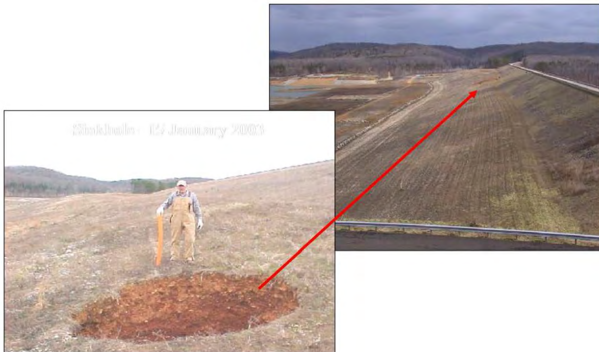
Figure 5.—Sinkhole through upstream impervious blanket.
