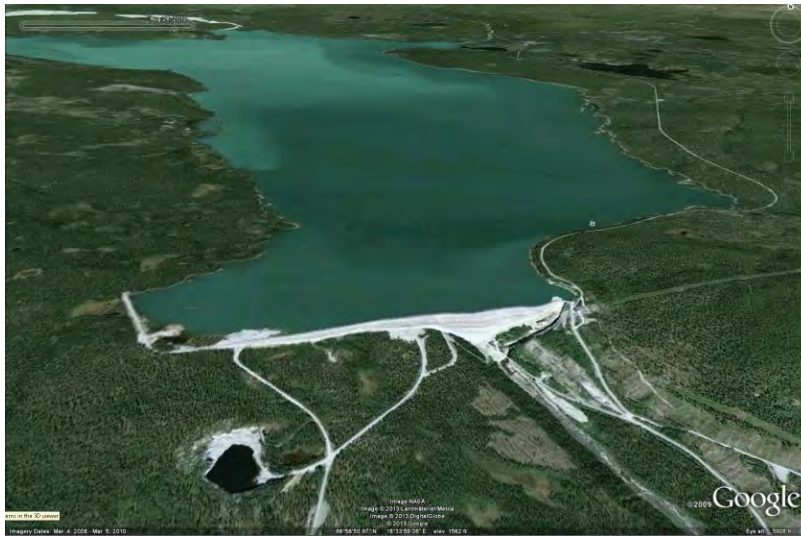
Figure 1.—The Seitevare Dam consists of a powerhouse, overflow spillway, main dam, and saddle dike. The right abutment was constructed on a glacial moraine.
