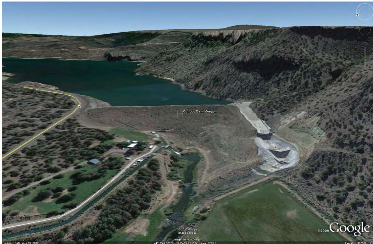
Figure 1.—Oblique view of Ochoco Dam, Oregon.
