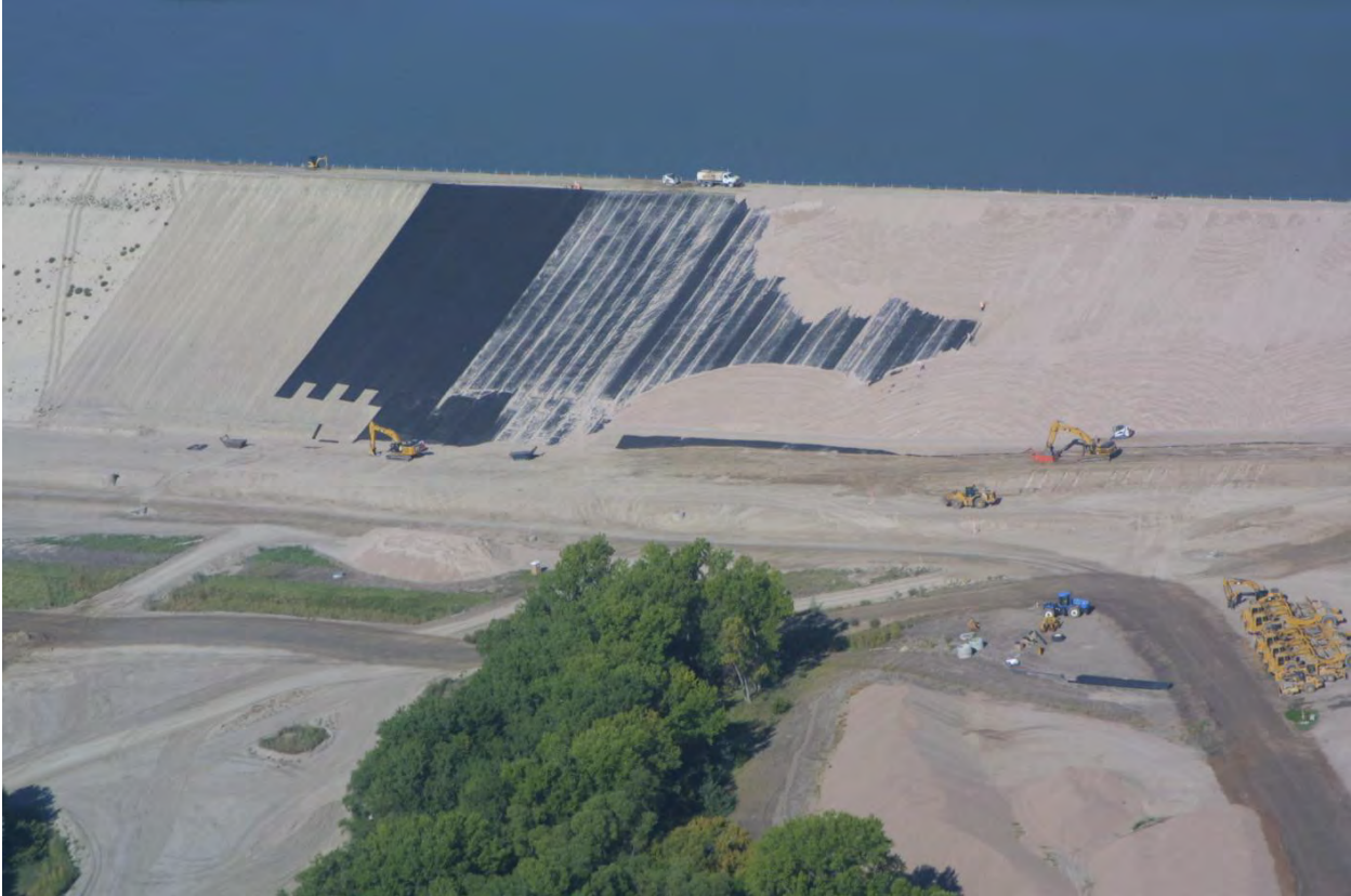
Figure 11.—Aerial photo of Red Willow Dam showing geo-net installation and protection with sand.
