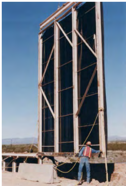
Figure 9.—Installation of geomembrane panel in the trench adjacent to previously placed panel.
