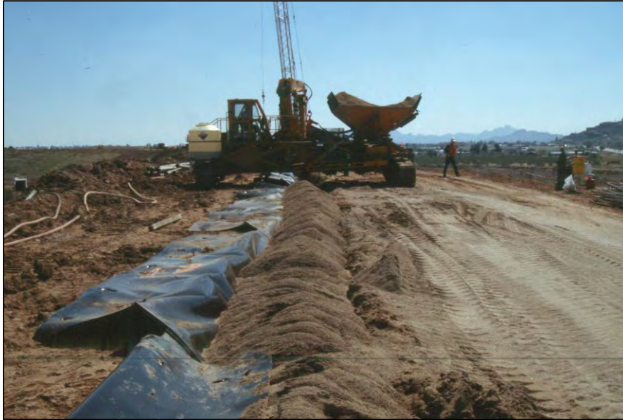
Figure 10-1.—Geomembrane cutoff with sand filter on Reach 11 Dike, Arizona. (Photo courtesy of Reclamation)
