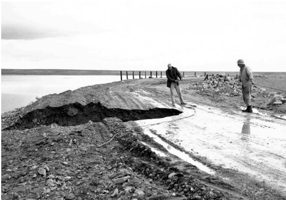
Figure 4a.—20-ft-diameter sinkhole on upstream side of dam crest. (Standing near the edge of a large sinkhole while hanging onto a rope is considered extremely dangerous and is not recommended.)
