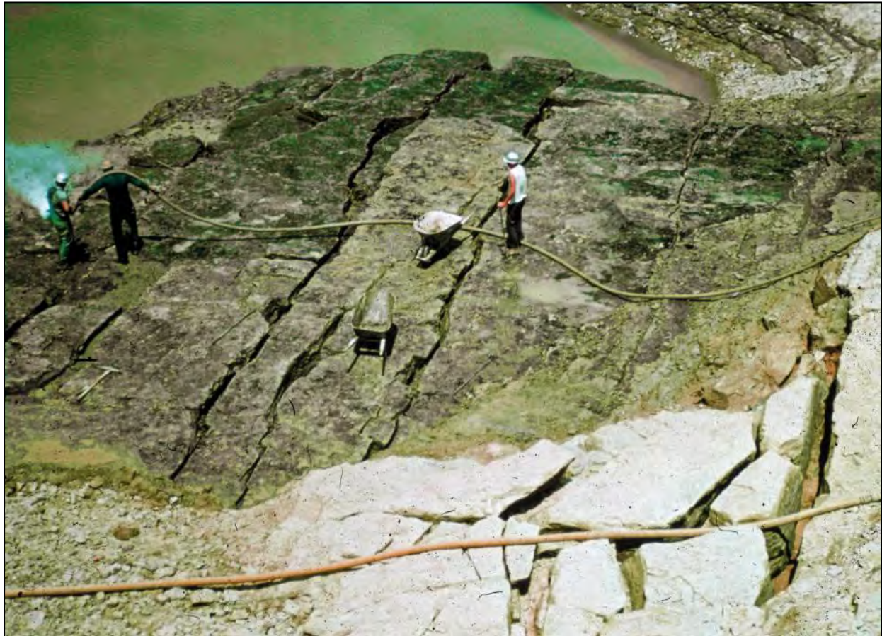
Figure 10-4.—Pressure washing joints and fractures in bedrock prior to dental grouting and covering with a blanket under the downstream shell of a dam. (Photo courtesy of NRCS)
