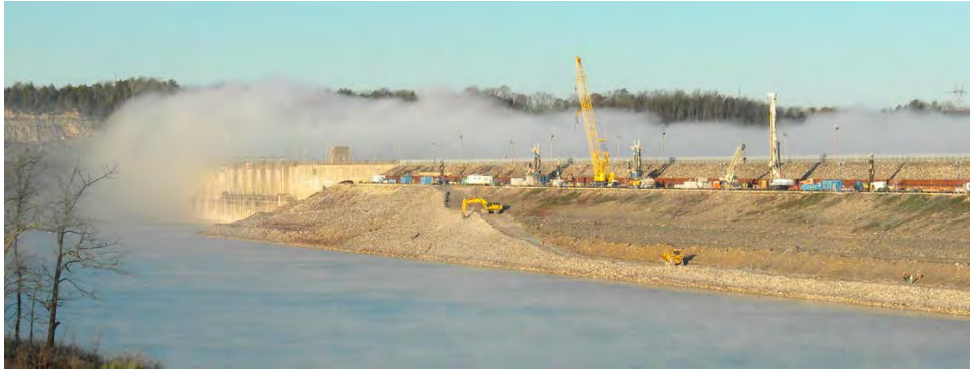
Figure 6.—View of working platform on upstream slope.
