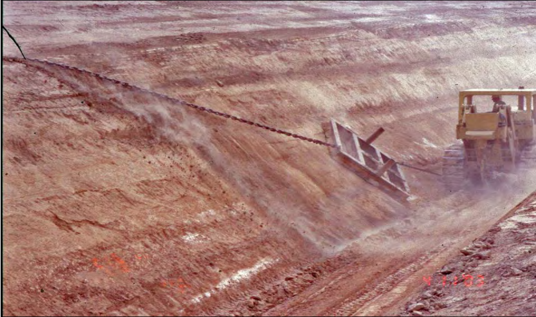
Figure 4.—Smoothing geotextile subgrade with metal frame, Olmitos-Garcias No. 2 Dam.
