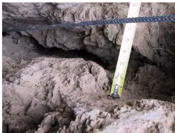
Figure 3.—Up to 5-in-wide cracks under holes.
