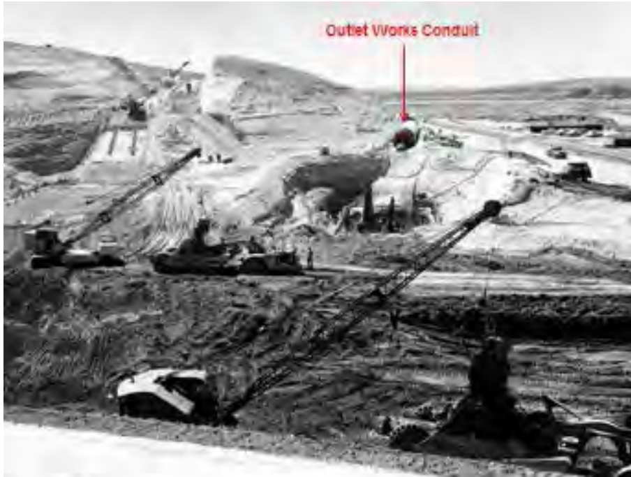
Figure 3.—Construction photo showing outlet works notched into firm Ogallala Formation.
