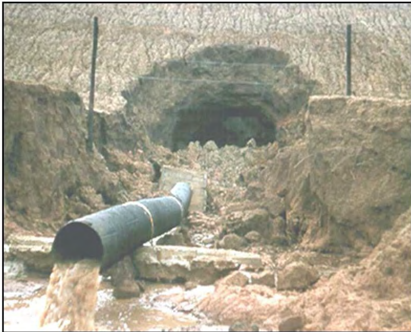
Figure 4-6.—Example of a dam that experienced gross enlargement, but the reservoir drained before erosion progressed to the point of crest collapse.
