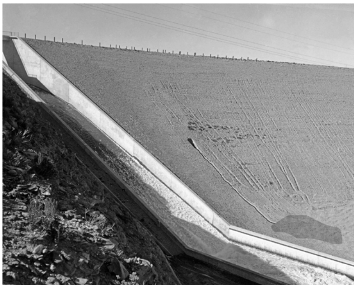
Figure 3.—First appearance of sinkhole, with drainage.
