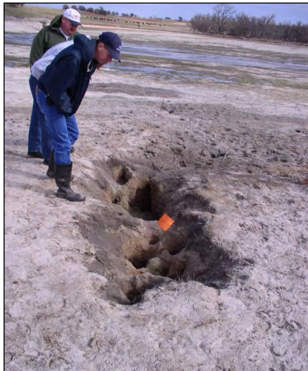
Figure 10-22.—Sinkhole in reservoir area of Little Washita No. 13, Oklahoma. (Photo courtesy of NRCS, Oklahoma)
