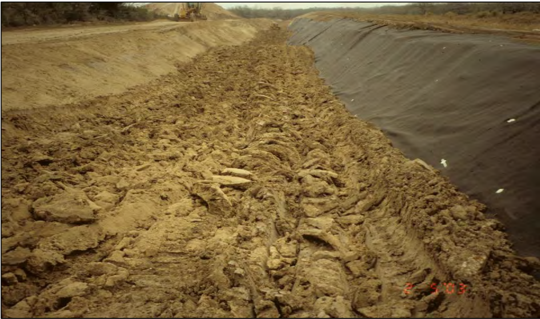
Figure 5.—Backfilling foundation trench, Olmitos-Garcias No. 2 Dam.
