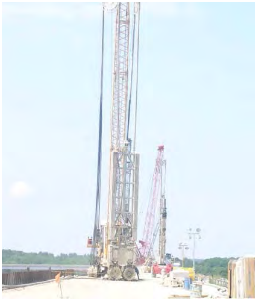
Figure 9.—Typical hydromill configuration.
