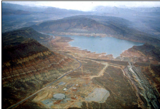
Figure 2.—The breach of the dike is located on the right limb of a large anticline where the rock outcrop extends beneath the dam in an upstream- downstream orientation.
