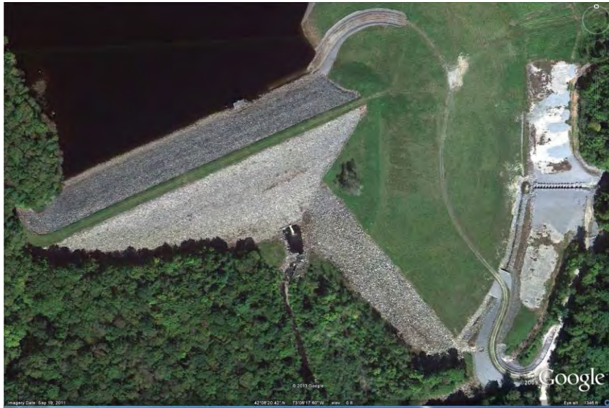
Figure 1.—Clam Lake Dam.
