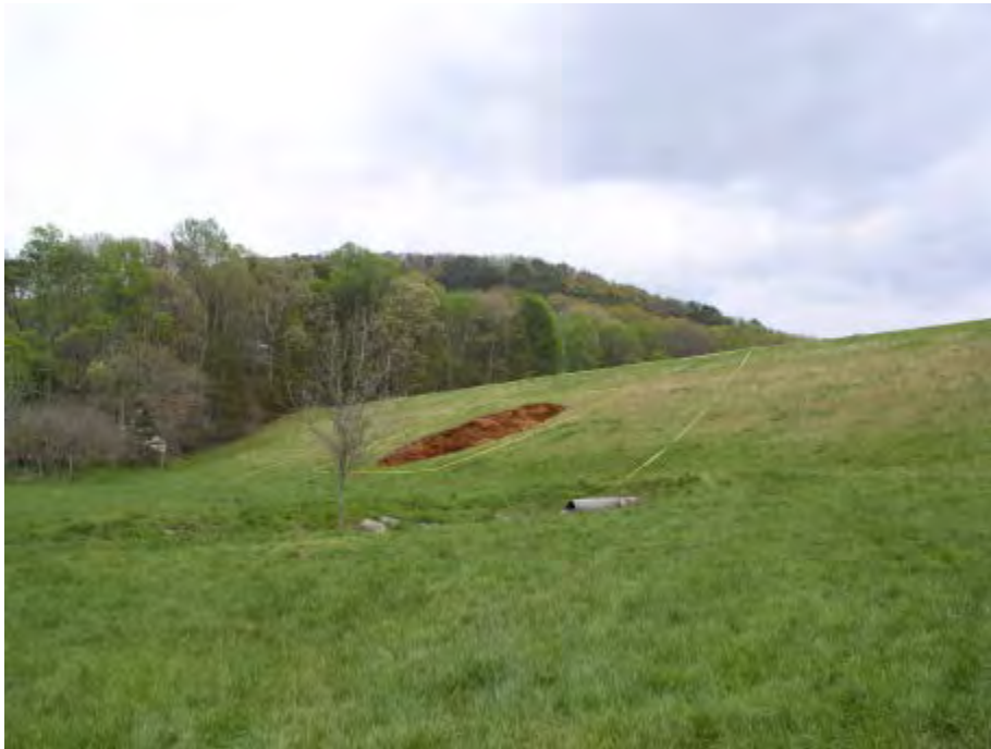
Figure 4-9.—Sallacoa Dam experienced a large sinkhole from internal erosion into a karst foundation.
