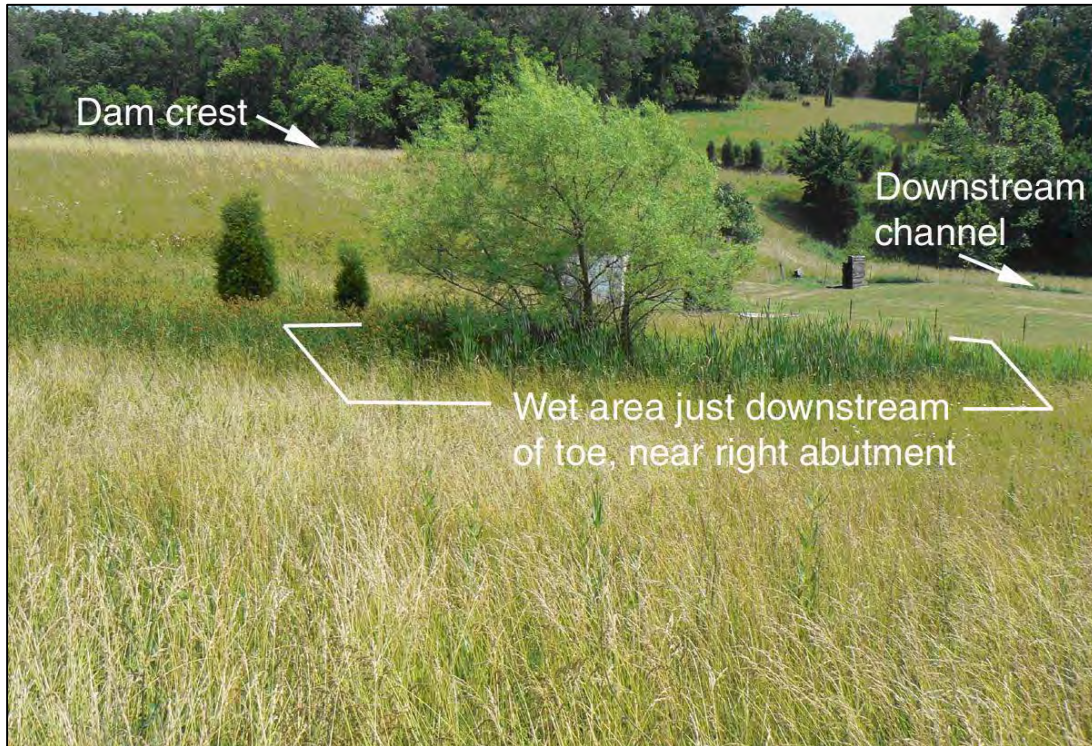
Figure 6-3.—Presence of phreatophytic vegetation (willow trees and cattails) in an established seepage discharge location approximately 200 feet below the downstream toe.
