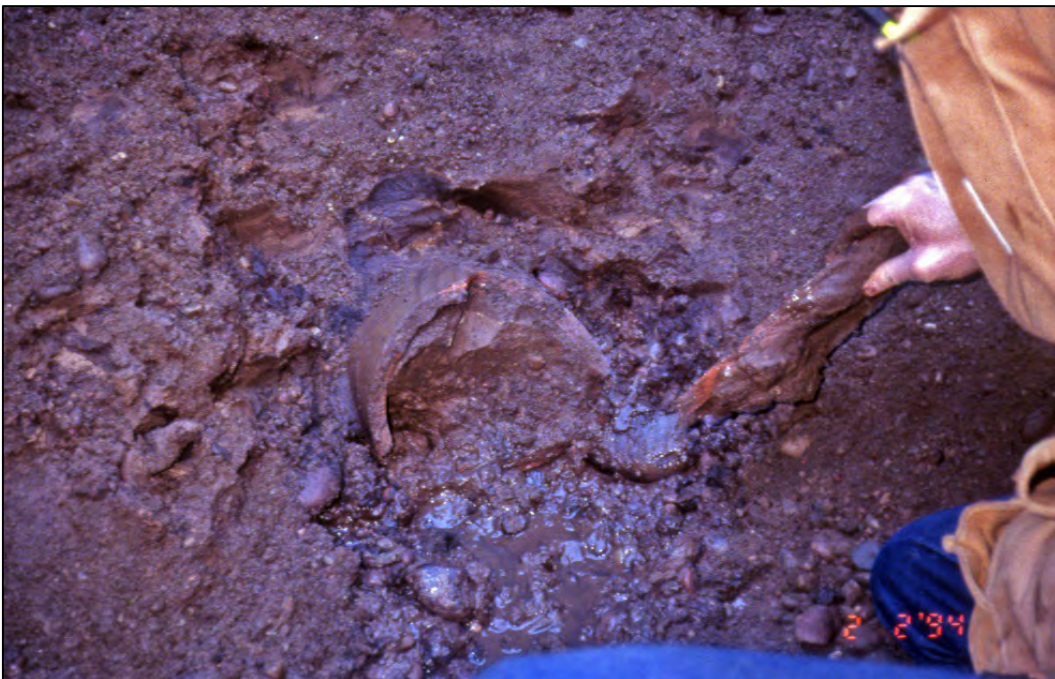
Figure 3-15b.—Excavation of the sinkhole shown in previous photograph revealed original toe drain below the sinkhole.
