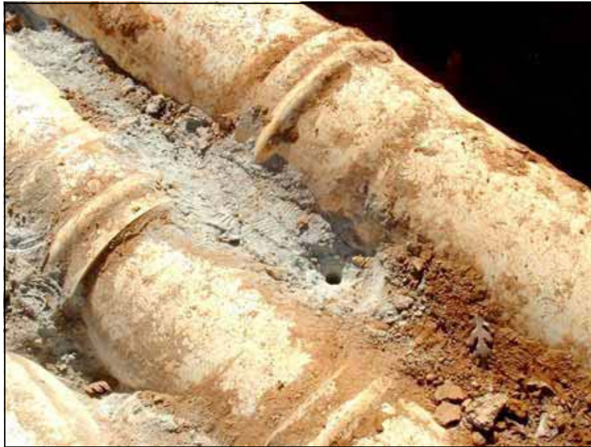
Figure B-14.—A small hole drilled through the concrete bedding between the siphons did not encounter voids under the concrete, even though the designer suspected that seepage was occurring directly under the pipes.
