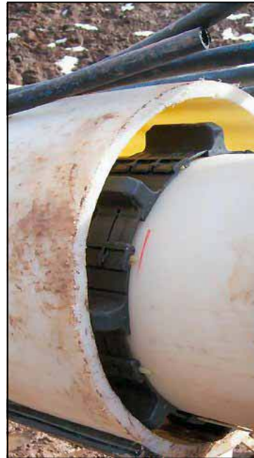
Figure 6. —Dual-wall containment HDPE pipe. A 14-inch diameter carrier pipe is being inserted into a 20-inch diameter containment pipe. Intermediate spacers are attached to the carrier pipe. Grout lines for grouting of the annulus between the existing conduit and containment pipe can be seen.
