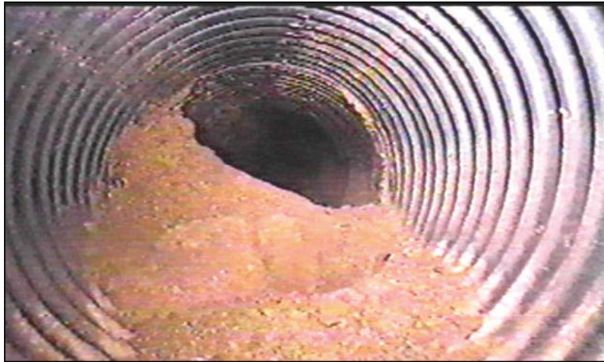
Figure 93. —This HDPE drainpipe has experienced joint separation allowing backfill materials to enter the drainpipe.
