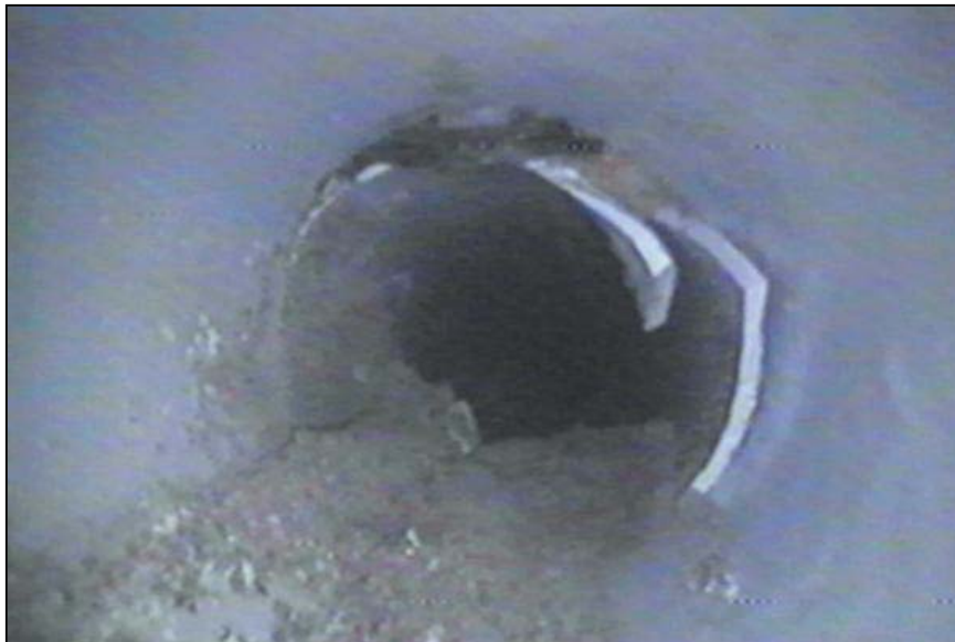
Figure 95. —PVC pipe used for toe drain has experienced transverse cracking. The cracking occurred during construction.
