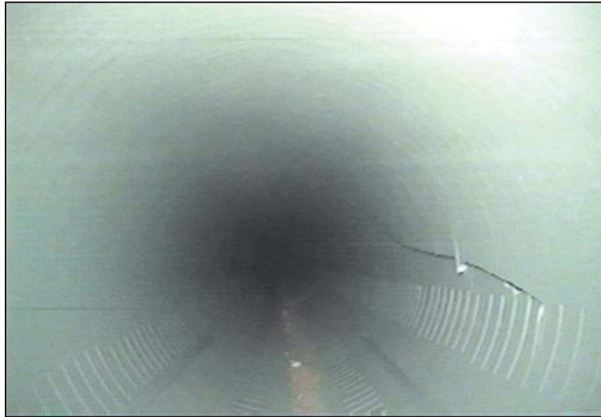
Figure 94. —Slotted PVC pipe used for toe drain has experienced longitudinal cracking. The cracking occurred during construction.
