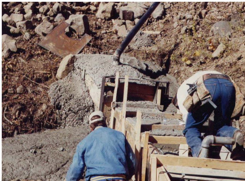
Figure B-16. —Looking upstream towards toe of dam: View of old box conduit and new downstream concrete encasement, during grout operation. Grout pipe is shown in top of photo.
