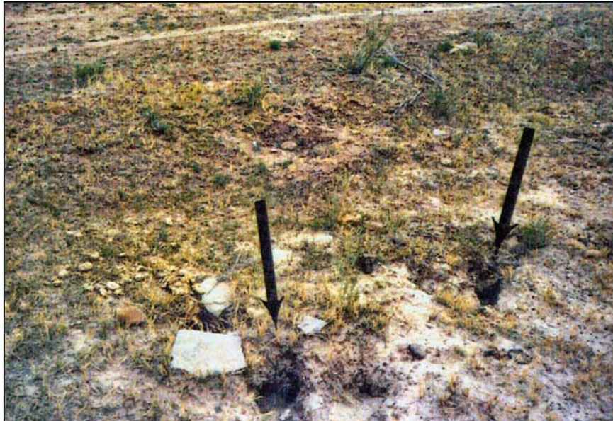
Figure B-5. —Erosional features typically associated with dispersive soils as seen at Ganado Dam. The common name for such features is “jughole.”
