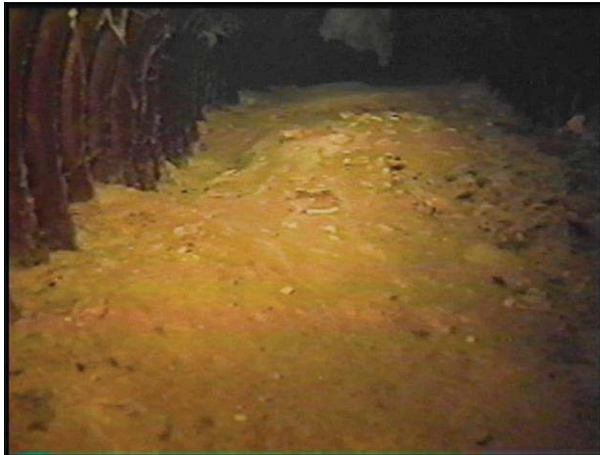
Figure B-2. —The typical amount of sediment deposition observed in toe drain during the November 2000 inspection.
