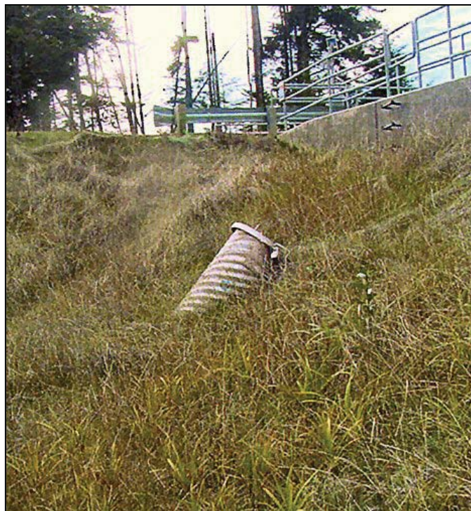
Figure 90. —Cleanout provides access to the drainpipe for CCTV inspection.
