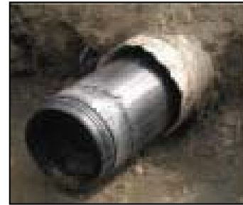
Figure 13. —Male end of snap joint.
