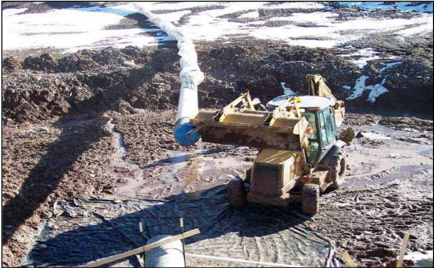
Figure B-24.—Guiding the 20-inch pipe into the upstream end of the CMP.
