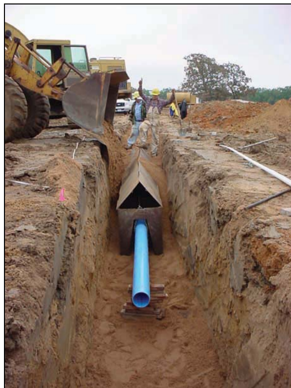
Figure 80. —A trench box or “doghouse” has been used to place material around drainpipes in vertically sided trenches in low hazard potential dams. Vertically sided trenches should not be used in significant and high hazard potential dam construction.
