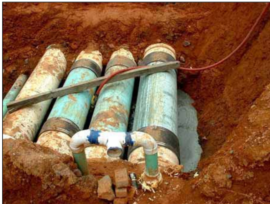
Figure B-15.—After removal of portions of the PVC siphons, it was determined that the original concrete bedding had been improperly placed, resulting in voids under the centers of the pipes. Portions of the siphons were replaced, and the bedding was replaced with a high slump concrete.
