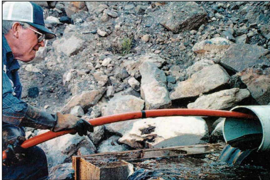
Figure 100. —Operator water jetting a drainpipe.
