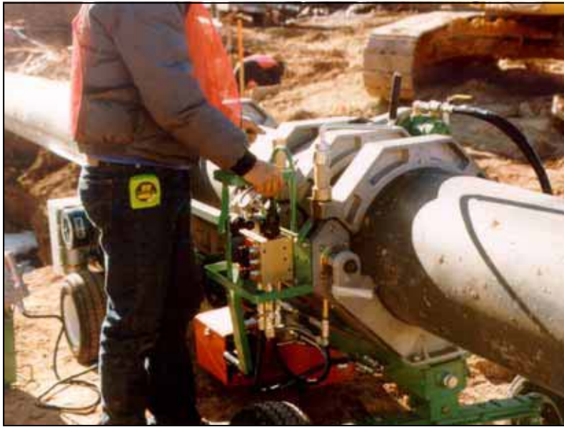
Figure 9. —HDPE pipe joint being butt fusion welded.
