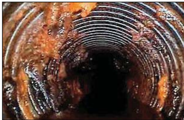
Figure 98. —Iron bacteria have partially blocked the perforations in this HDPE drainpipe. Note that the only open perforation passing seepage is in the lower left corner of figure.
