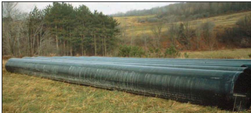
Figure 5. —Solid wall HDPE pipe to be used for sliplining of an existing outlet works conduit.
