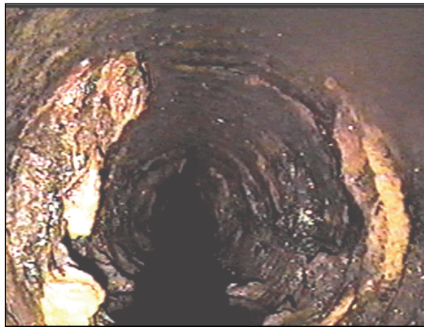
Figure 97. —Calcite deposits have formed at joints and perforations in this HDPE drainpipe.
