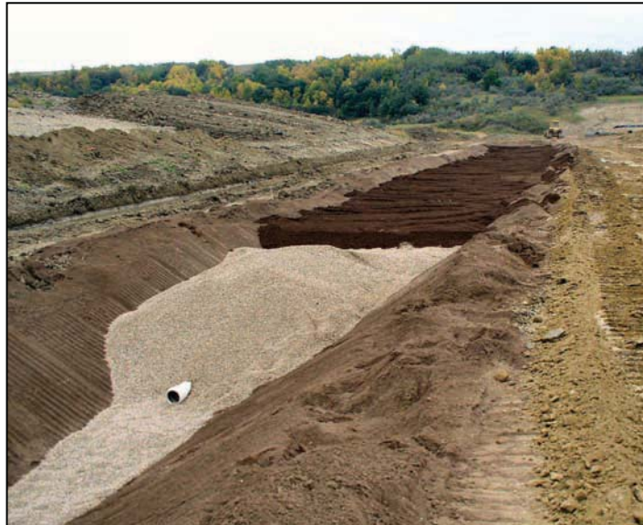
Figure 79. —Filter material being placed over drain material.
