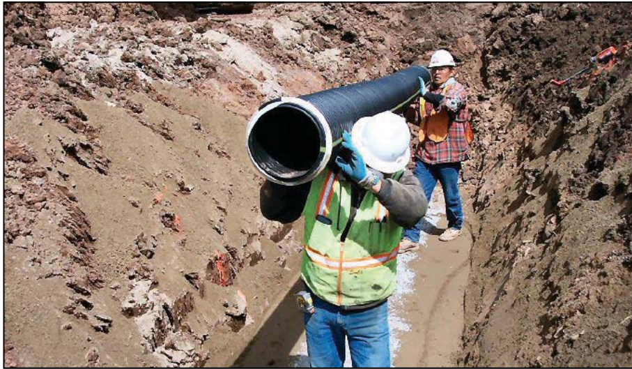
Figure 1.—Plastic pipe is lightweight, which facilitates installation.
