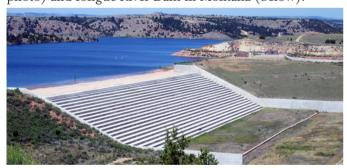
The most common use of RCC for overtopping protection of a concrete or masonry dam is to provide a massive buttress for the structure to improve sliding stability. RCC may also be used to protect the dam foundation from erosion and headcutting from an impinging jet, but would not lend itself to the protection of steep abutments.
