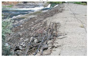
Riprap has long been used for embankment dams to prevent rill erosion of slopes due to surface runoff and to prevent wave erosion at the interface between embankment slopes and standing water. Riprap has been widely used in arid areas and on steeper embankment slopes (up to about 1.5:1) where vegetation is difficult to establish and maintain.
