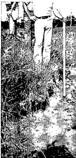
Right: Beaching of an upstream slope.
