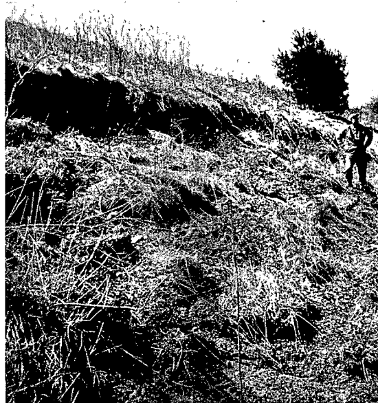
Left: Scarp - The exposed slope above a slide.
