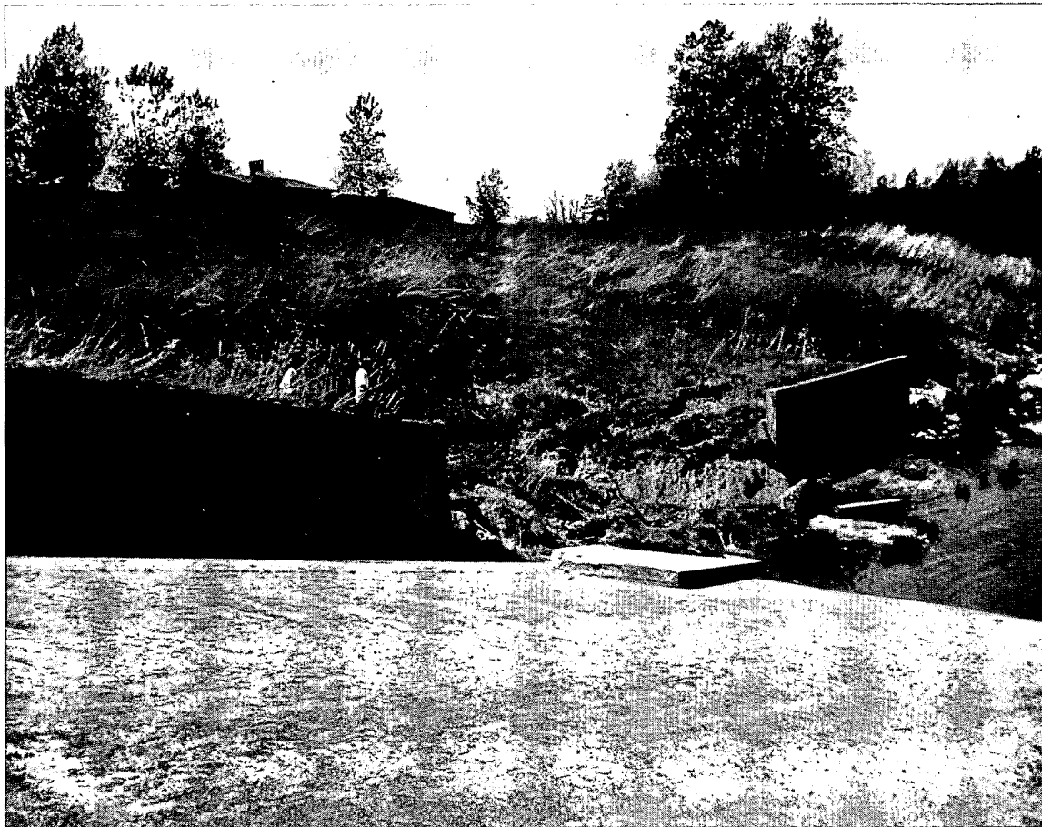
Collapse of a spillway wall section.
