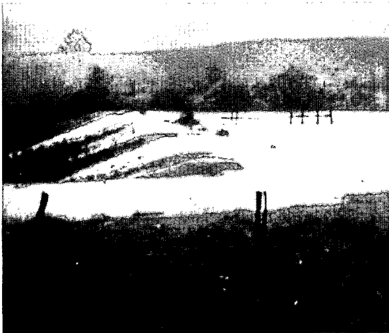
A dam being overtopped.
