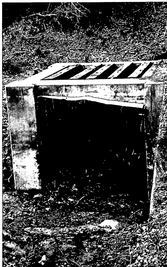
TRASHRACKS ON PIPE SPILLWAYS
