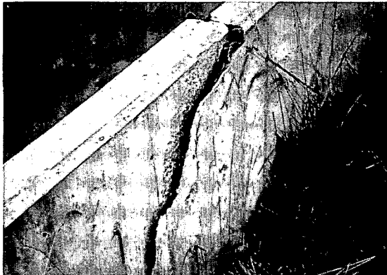
Right: Structural crack caused by wall movement.
