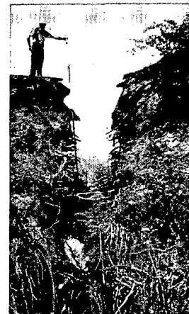
Left: Tree roots in an embankment.
