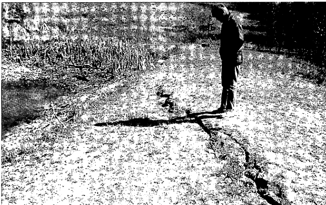
Longitudinal crack.
