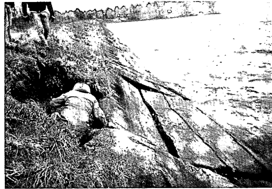
Lower left: Large void beneath slabs of concrete.
