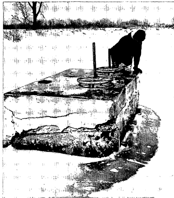
Left: Concrete deterioration caused by weathering.
