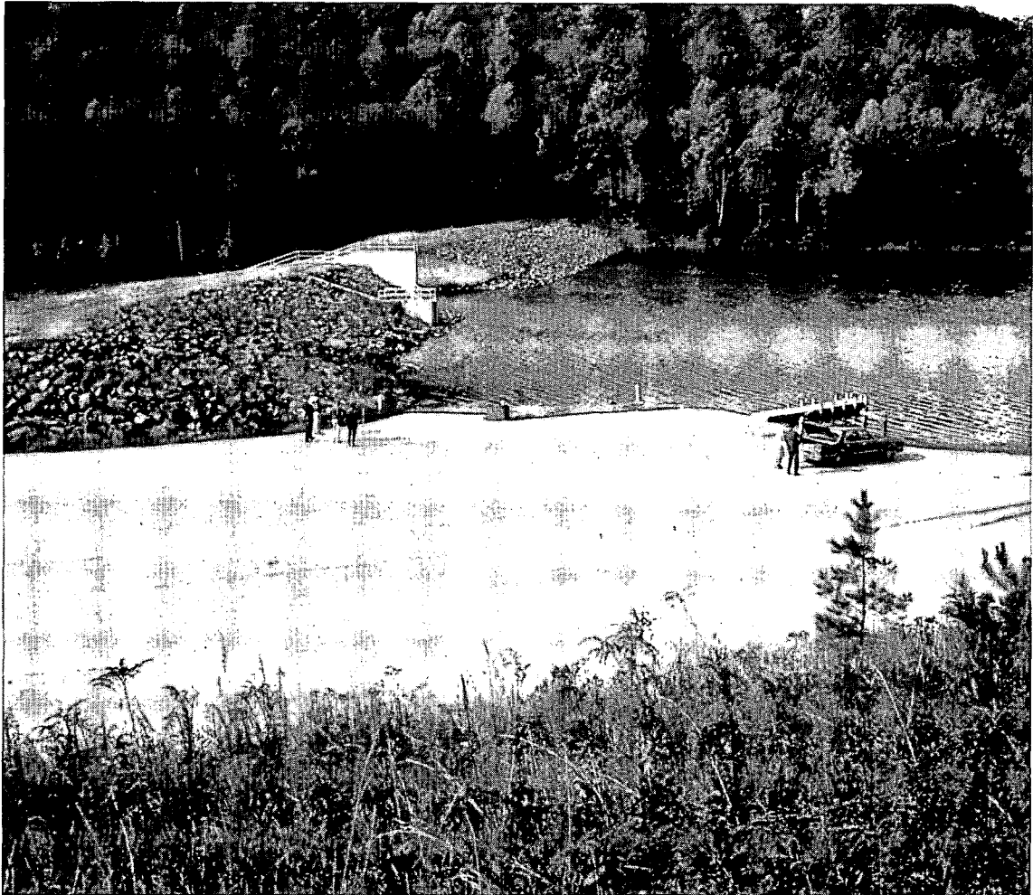
An emergency spillway being used as a parking lot and boat launching ramp.
