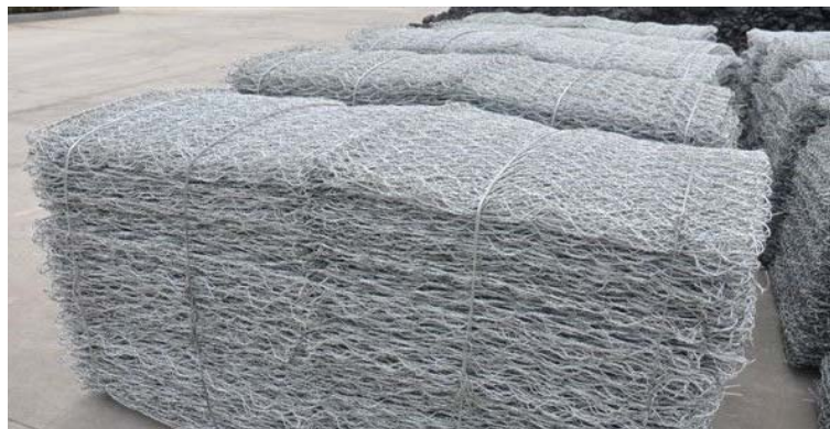
Figure 5-1.—Example of gabion baskets delivered to the project site (Reclamation, courtesy of Chris Ellis).
