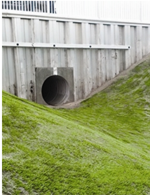
Figure 6.1.—HydroTurf™ Outfall Structure with St. Johns River Water Management District in Florida (Courtesy of Watershed Geo, all rights reserved).
