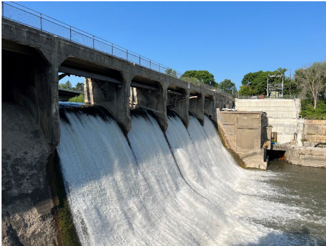
Figure 4 Rapidan Dam (Photo Credit: Barr Engineering Co.)
