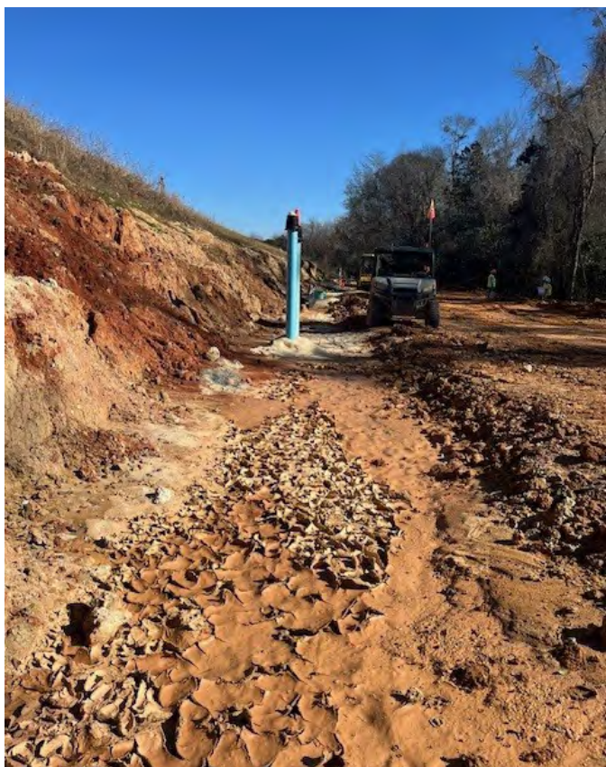
Figure 4 Relief Trench Midslope of Embankment
