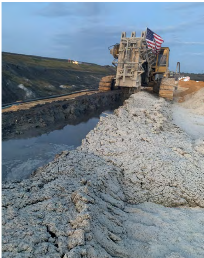
Figure 3 Trencher With Soil-Mixing Blade in the Trench
