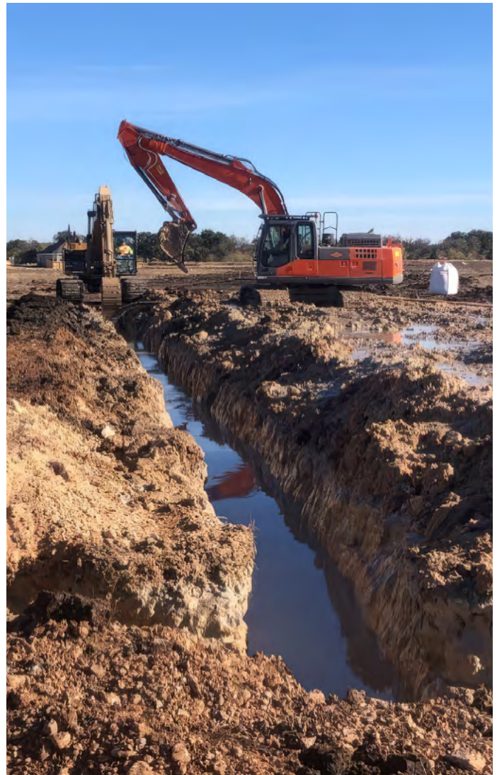
Figure 5 Slurry Trench Method
