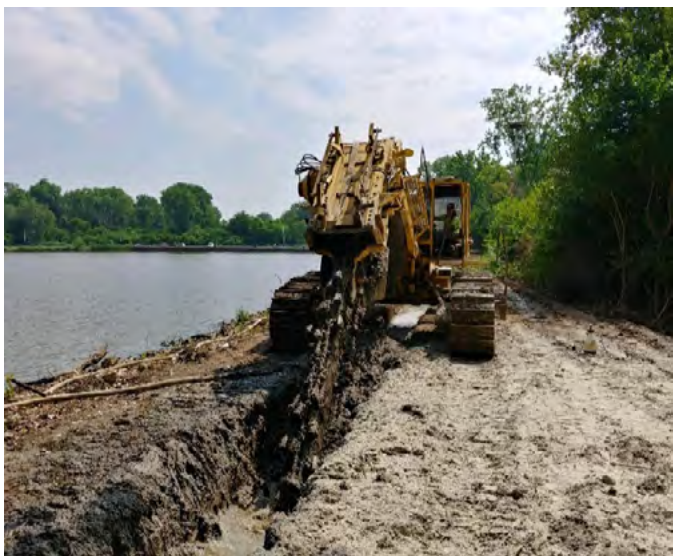
Figure 2 Trencher With Soil-Mixing Blade Visible Halfway Out of Trench
