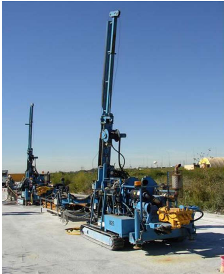
The use of a hard-surfaced work platform and state-of-the-art drilling equipment make it possible to more accurately construct grout curtains of greater depths.
