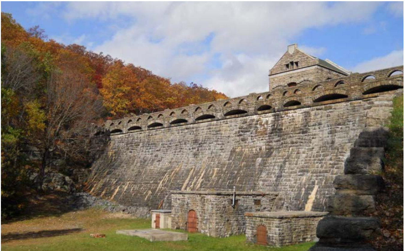
Figure 2. Masonry section of Lake Scranton Dam.
