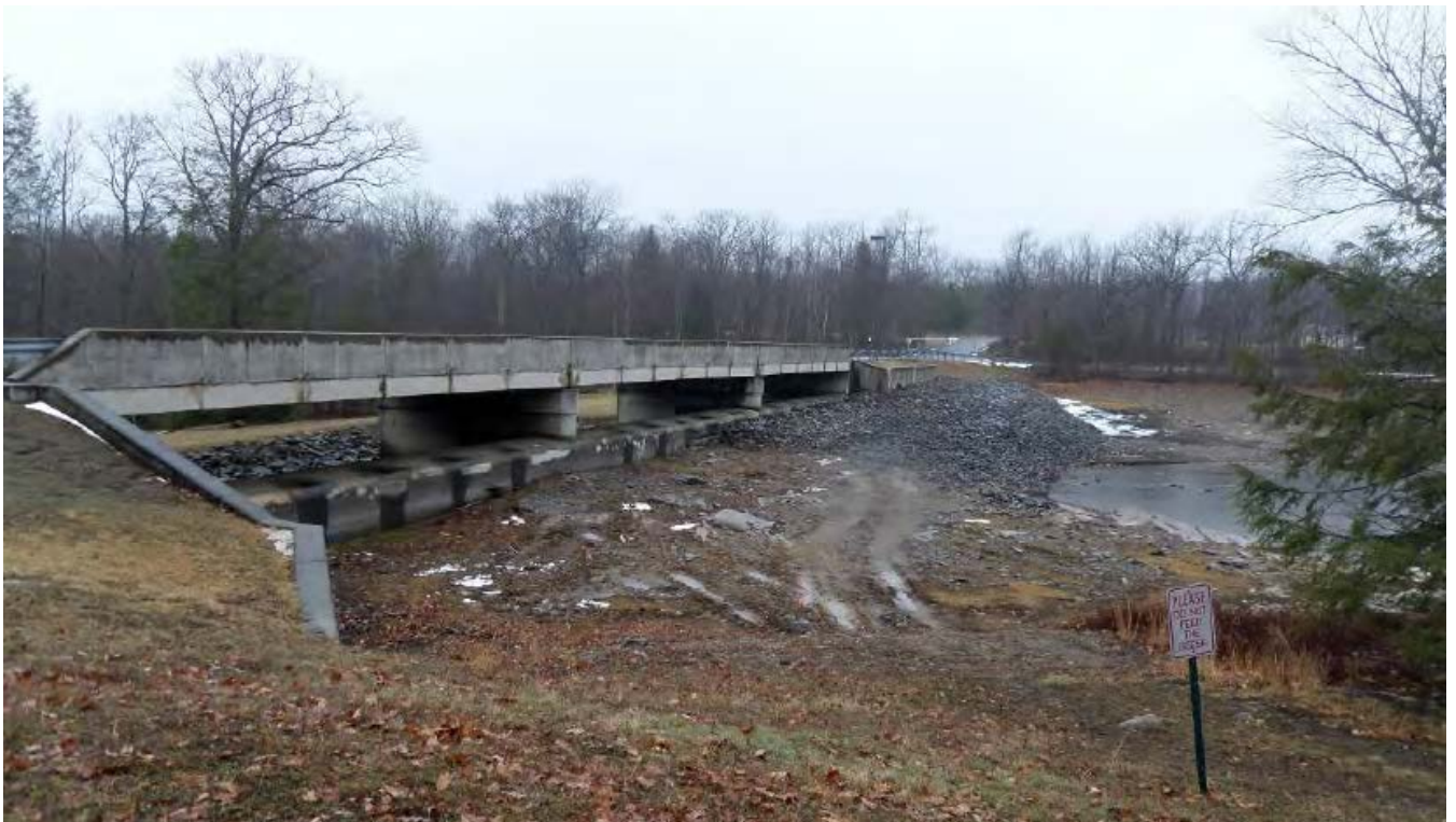
Figure 3. Existing ogee crest spillway at Lake Scranton Dam.
