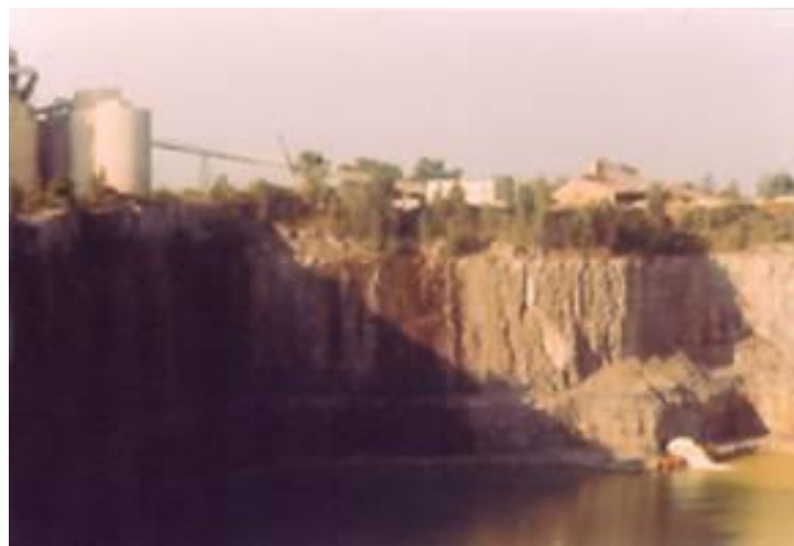
Sudden development of large flow (over 30,000gpm) through karst into the base of an operational quarry. Nearby river provides infinite source and driving head of over 300-feet.
