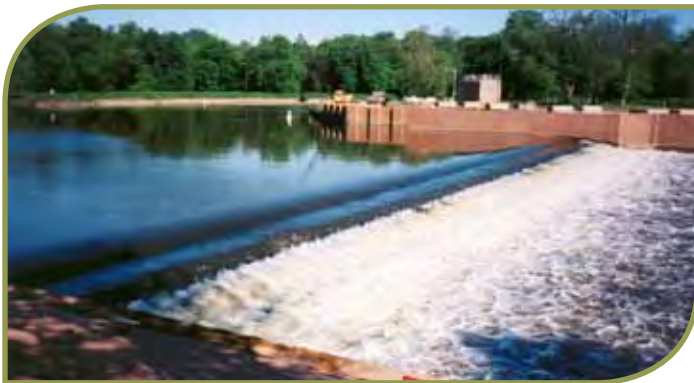
Figure 7. Island Farm Weir stepped spillway modification.
