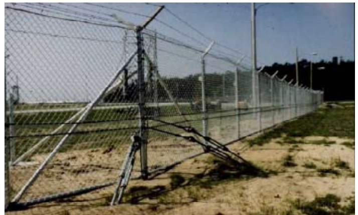
Figure 2: Anchored Fence
