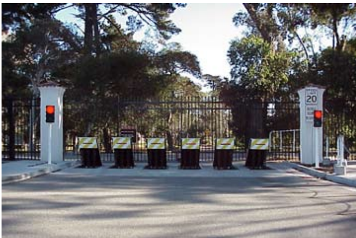
Figure 1: Use of Active and Passive Barriers
