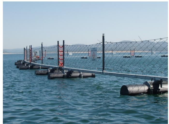
Figure 4: Net Boat Barrier
