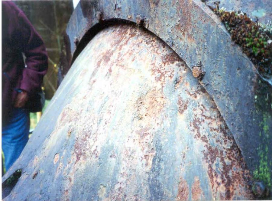
**Photo 2** - Valve stuck in the closed position due to lack of maintenance.
