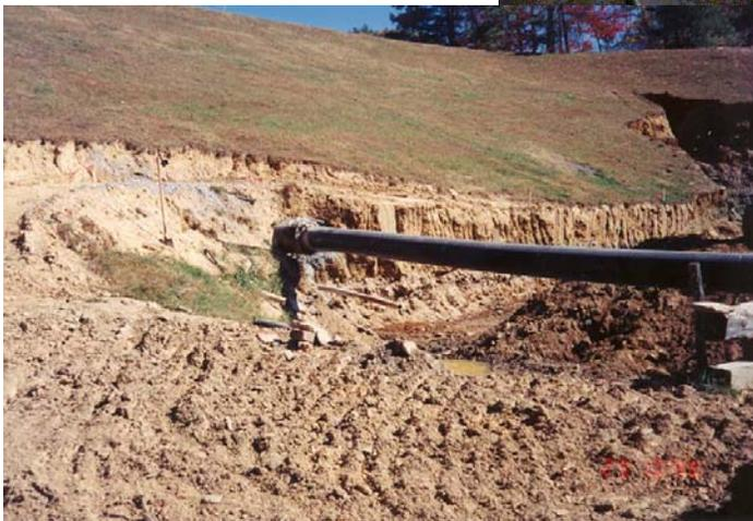
The liner will typically have a roughness value of approximately  $\frac{1}{2}$  of the corrugated metal pipe. When designed and installed properly, the slipline technique will add additional years of service life to the existing pipe conduit spillway. A sand diaphragm drain is typically installed around the downstream portion of the existing conduit to limit the potential for soil piping as the CMP eventually corrodes and deteriorates.
