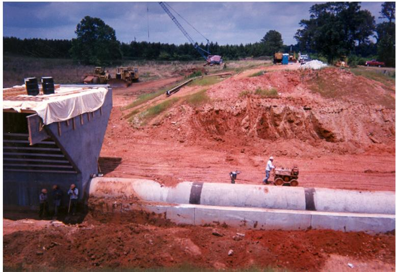
Removing and replacing the existing conduit typically offers the most thorough rehabilitation option for impaired conduits through dams, although this option can be cost-prohibitive.
