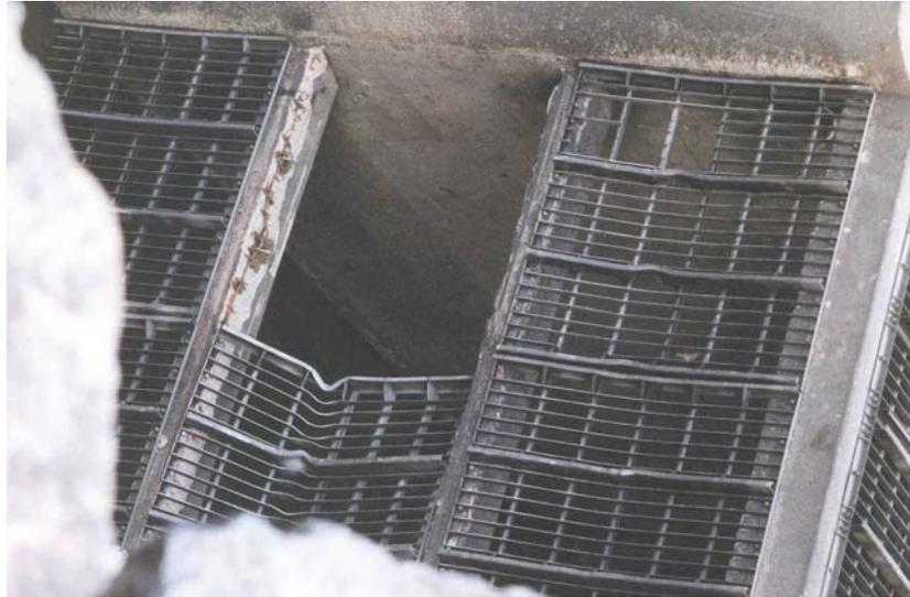
**Photo 1** – Collapse of Trash Rack at Yard's Creek Dam.
