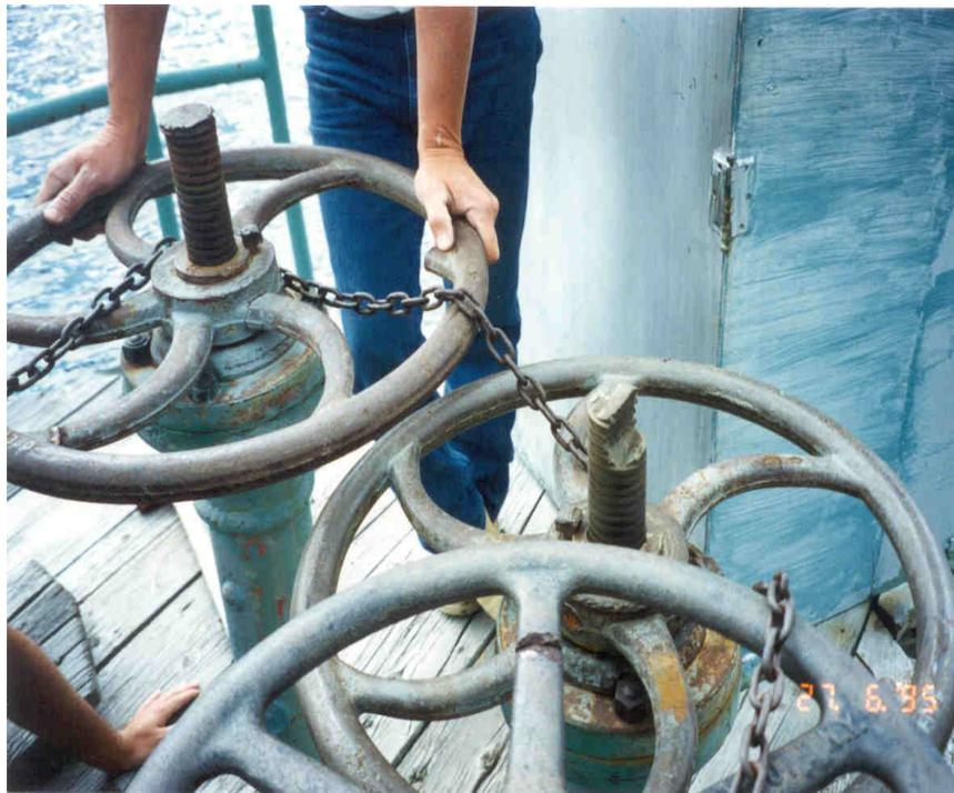
**Photo 3** – Broken Gate Operators at an Intake Tower.
