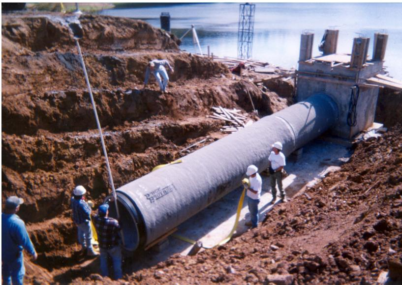
location of the upstream pipe invert (entrance to the pipe) relative to the hydraulic grade line. Subatmospheric pressure conditions, that can accompany entrance conditions for steep pipes should be avoided. Also, the conduit invert should be a minimum depth of 1.5 diameters below the pool elevation to avoid the capture of air due to surface water drawdown, and associated “slugging” under full flow conditions.
