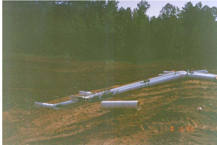
traditional pipe-and-riser spillway systems, generally results in a lake that will fluctuate more as a result of the inherent inefficiency of the siphon until priming occurs. Siphons prime with a head or water surface elevation between 1 and 1-1/4 times the diameter of the siphon above the siphon invert. Once a siphon primes, there is very little increase in outflow as the lake surface rises.
