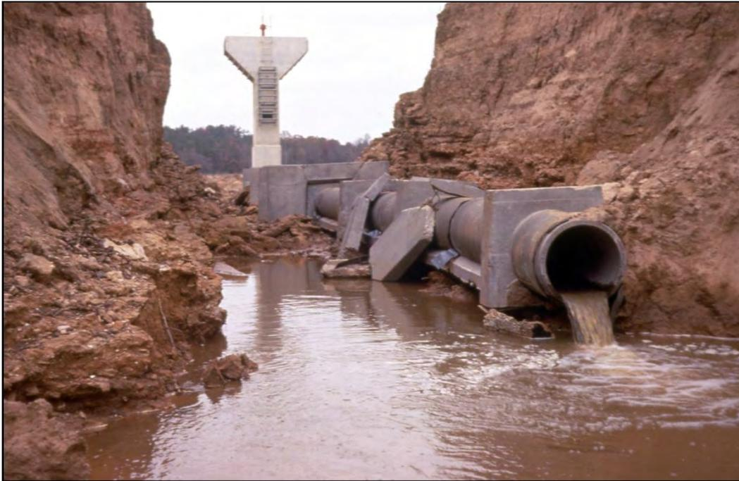
**Figure 2-5. Embankment dam breached after piping along the conduit. The view is upstream. Note pre-cast concrete pipe placed on a concrete cradle and the use of seepage collars (Photo credit NRCS).**
