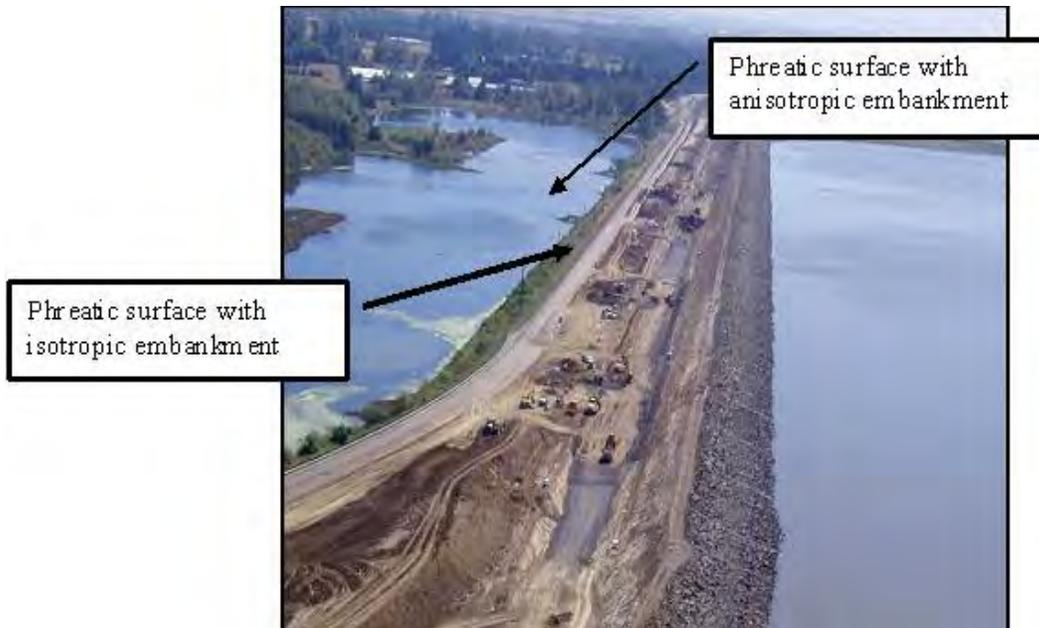
Figure L-31-2.—Foundation trench drain placed inside the downstream embankment section in an attempt to both collect foundation seepage and lower the phreatic line. At Fern Ridge, this dual function was not successful.
