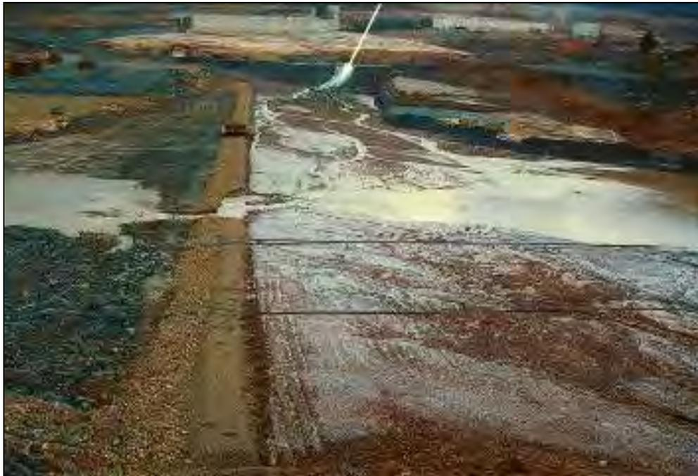
Figure 7-25. Surface water contamination of a chimney filter.
