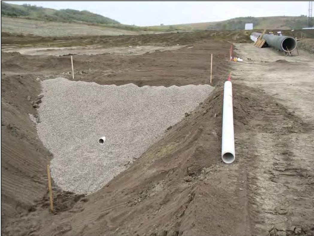
**Figure 2-14. Trapezoidal foundation trench drain at toe of embankment. Coarse inner filter surrounds perforated PVC collector pipe and fine filter provides filter compatibility with foundation soils.**
