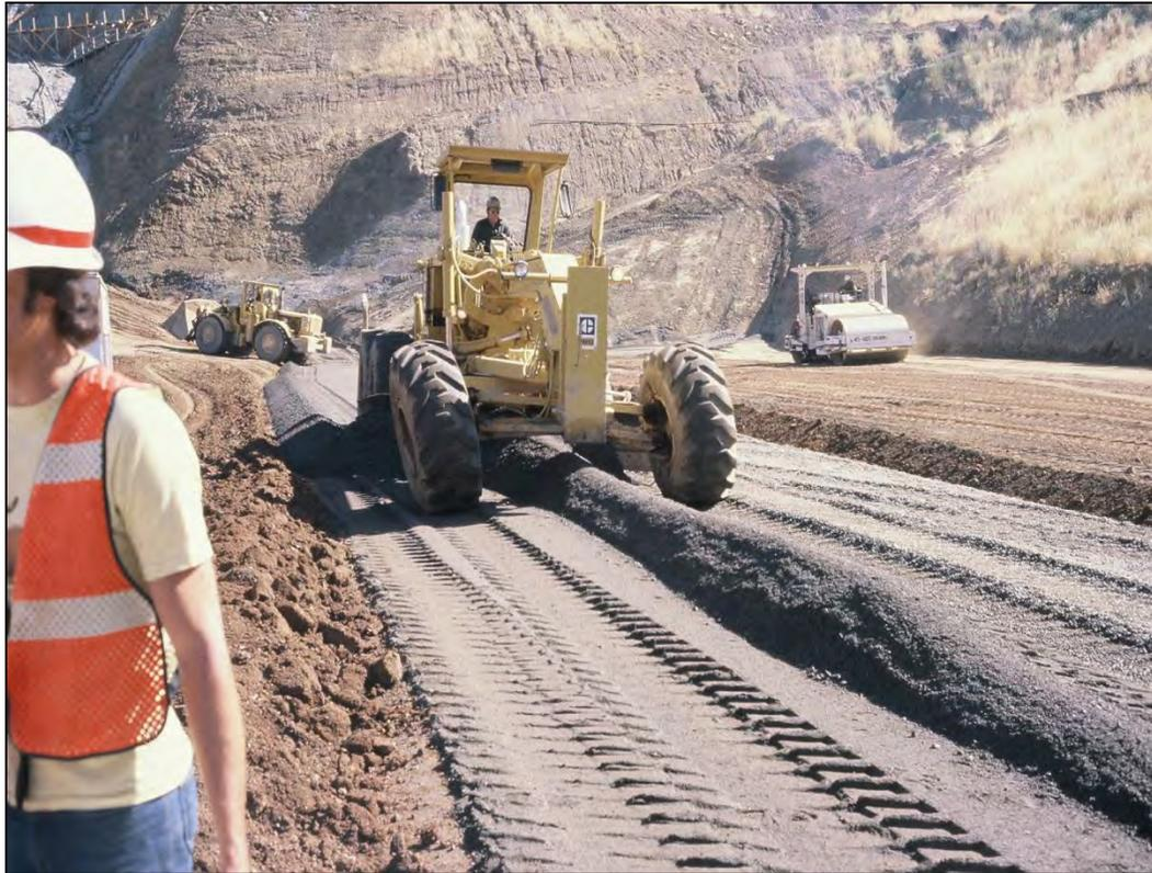
Figure 7-13. Spreading sand filter material.
