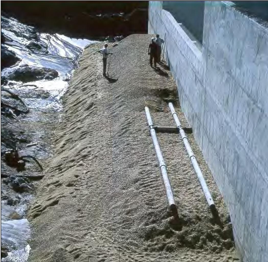
**Figure 2-7. Filter and drainage zones to provide pressure relief and drainage of backfill next to training wall for a spillway chute. One individual is standing on top of the sand layer (Photo courtesy of NRCS, Texas).**
