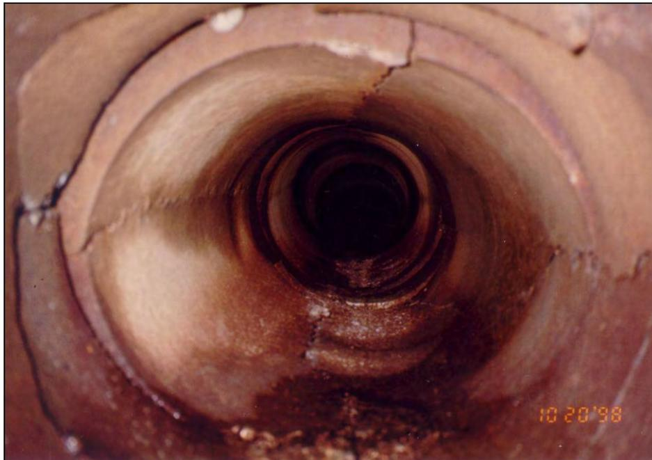
Figure 2-17. Interior view of a reinforced concrete pipe from the 1950s. Note that the pipe is overstressed, and cracks have formed at the crown and spring line. The pipe has also deformed to an oval shape. In the foreground, a joint can be seen and sand that passed through the joint.
