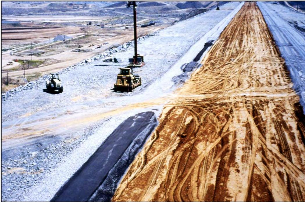
**Figure 7-26. Haul road crossing of a chimney filter and drain.**
