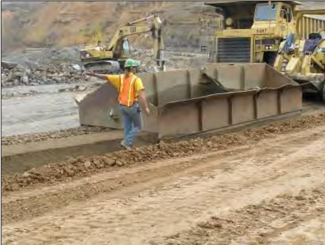
Figure 7-17. Towing spreader box.
