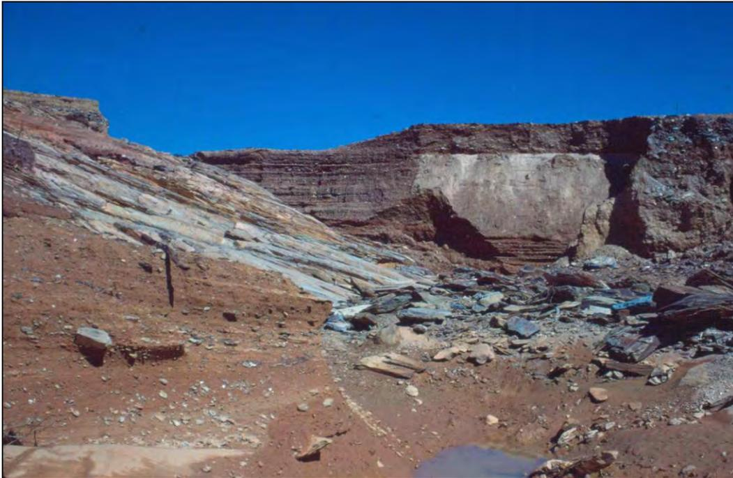
Figure E-3. Breach in left abutment viewed in upstream direction. Right abutment is to left foreground. Overtopping flow washed the embankment and overburden down to clean rock.
