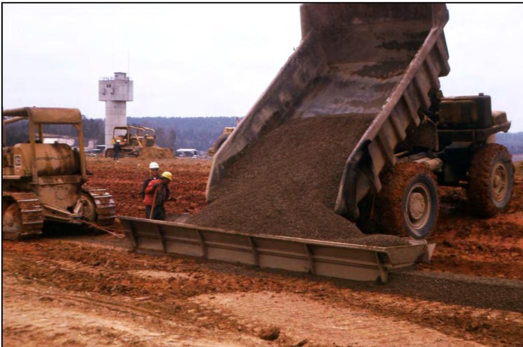
Figure 7-16. Dumping into spreader box.
