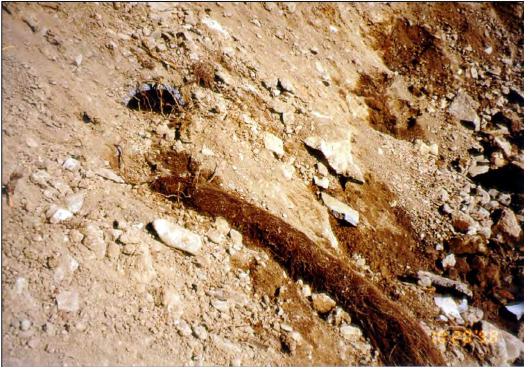
**Figure 2-19. During modification of a dam, this toe drain pipe was exposed during excavation. The pipe was completely clogged with the root ball shown in the foreground. It was noted that a tree was growing over the toe drain, and the drain was probably the water source in this arid region of central Oregon.**
