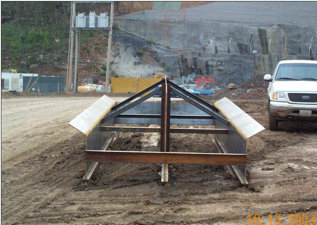
Figure 7-15. Double-bin spreader box.
