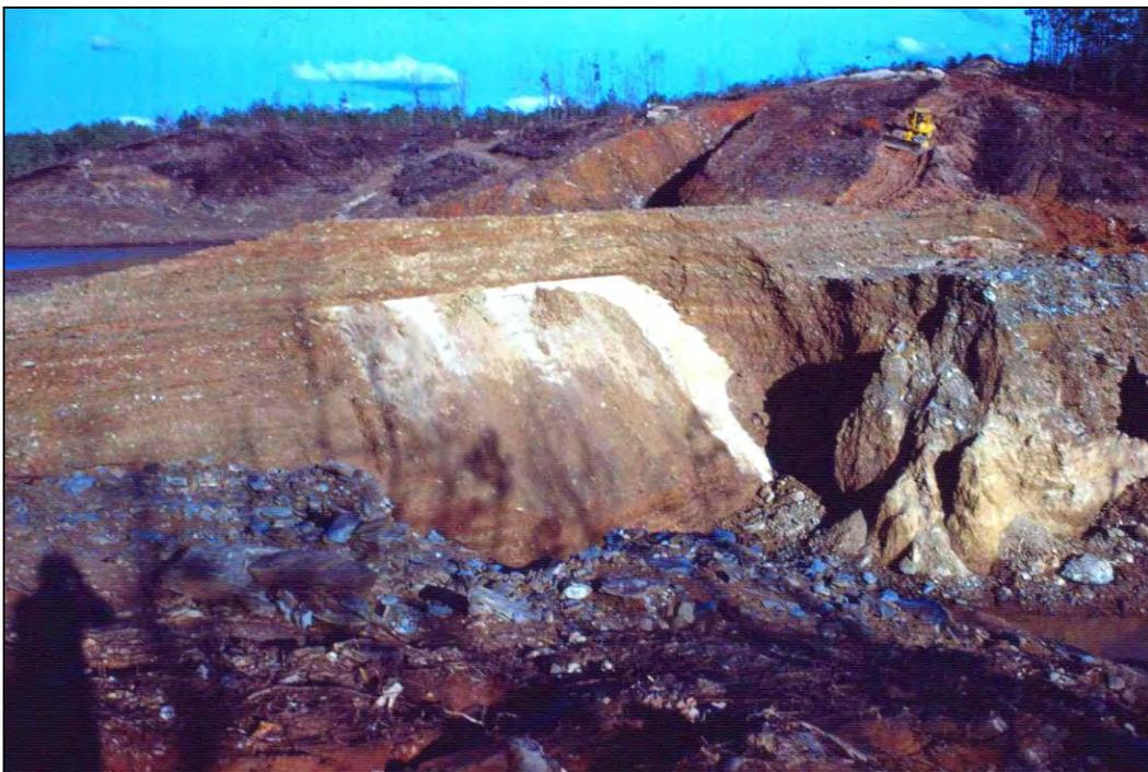
Figure E-6. Breached portion of dike in left abutment viewed upstream. The lighter color is remnant of a chimney filter.
