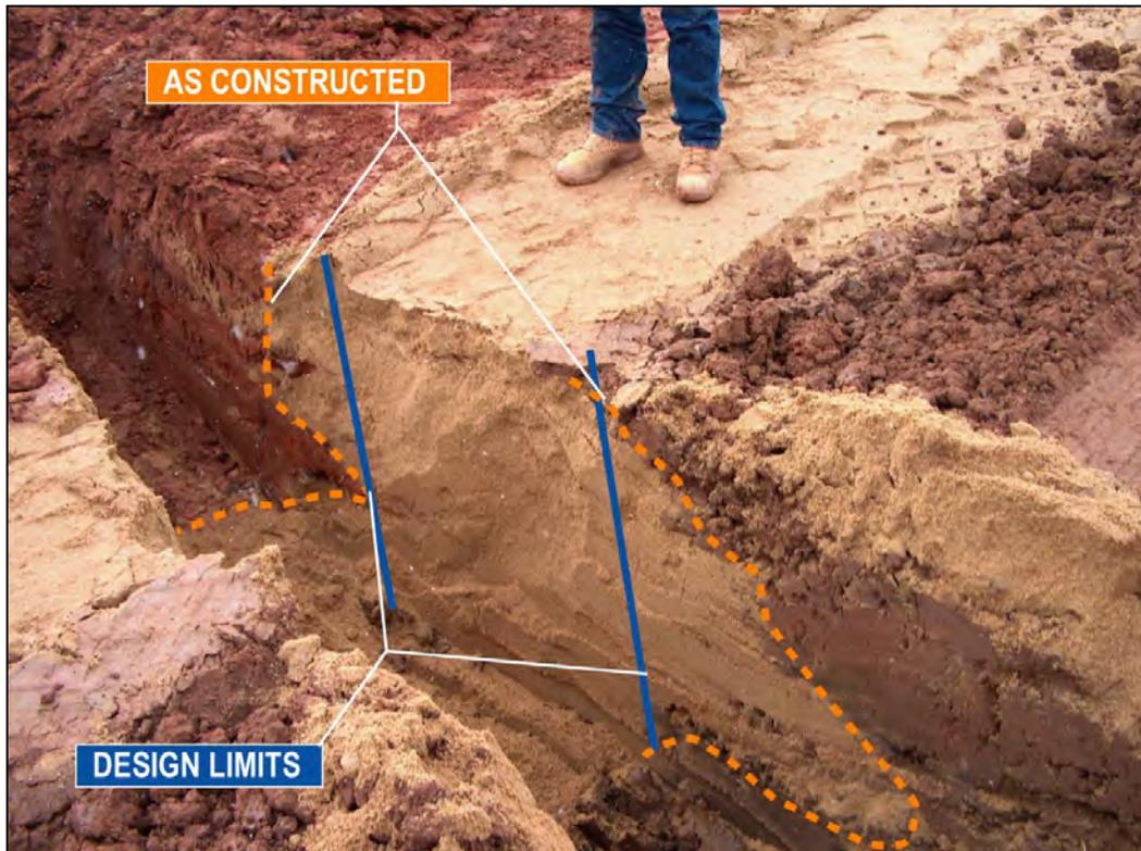
**Figure 6-4. “Christmas tree” effect in a sloping chimney filter.**
