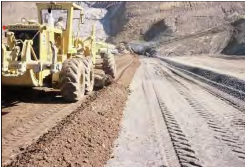
Figure 7-3. Windrowing impervious material adjacent to a filter/drain.
