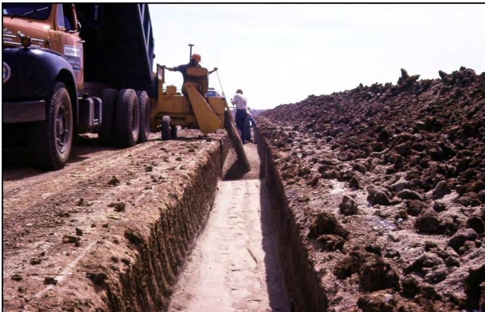
Figure 7-6. Trenching method – backfilling trench.
