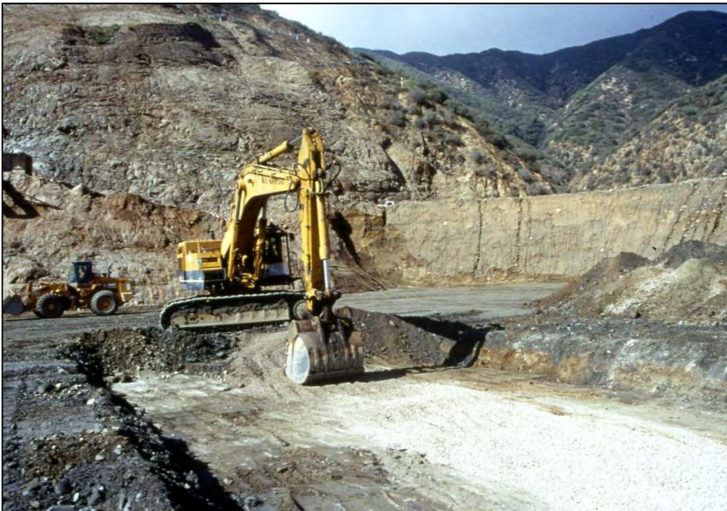
**Figure 7-27. Excavation of filter material under equipment crossing.**
