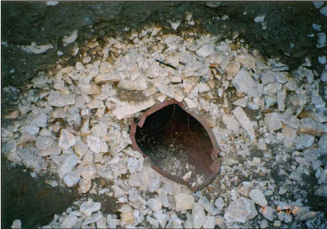
Figure 2-16. Clay tile pipe surrounded by gravel-size material. Note mechanical pencil for scale. Surrounding the gravel is a mixture of silt and sand backfill that does not meet filter criteria for the gravel. Seepage enters the pipe through joints between pipe segments. The silt and sand can erode through the gravel backfill and enter the pipe through the joints.
