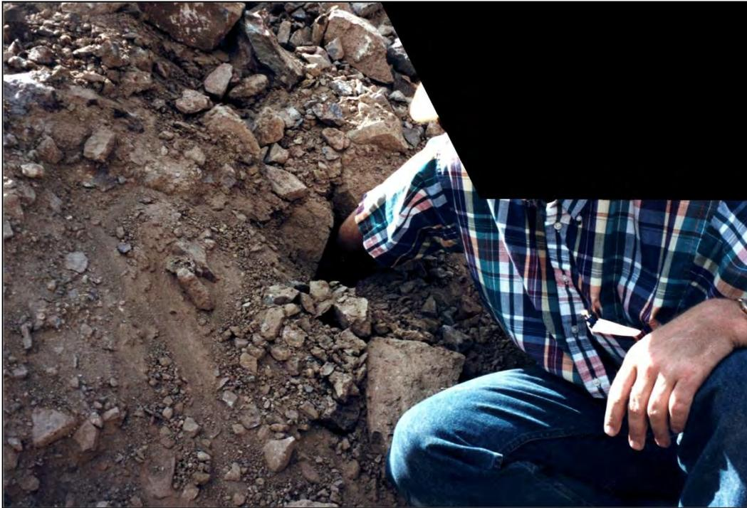
**Figure 6-6. Open work present in the right abutment foundation of Ochocho Dam. The abutment consists of landslide debris.**
