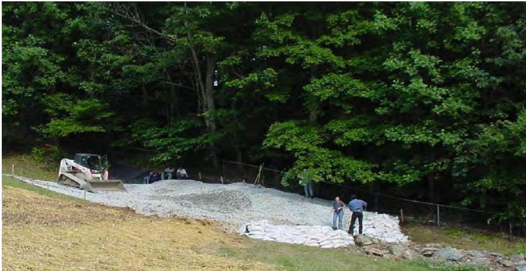
**Figure L-26-2. Gravel drain being placed over seepage area.**
