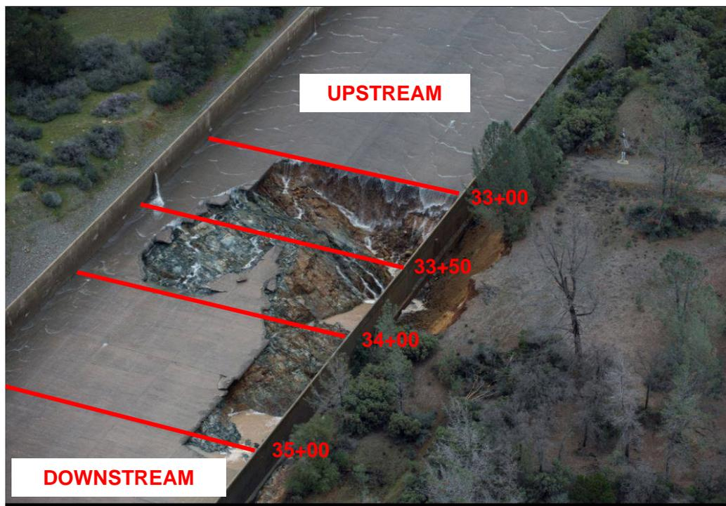
***Update on Physical Factors Evaluation for Service Spillway Chute Failure*** – While there are numerous physical factors that contributed to the failure, which the IFT has studied in detail, the IFT has focused on the critical factors that it believes likely played the most significant roles in the failure of the service spillway chute. As noted above, the IFT had previously prepared a list of potential physical factors under consideration, and now has a more refined view of these factors.
