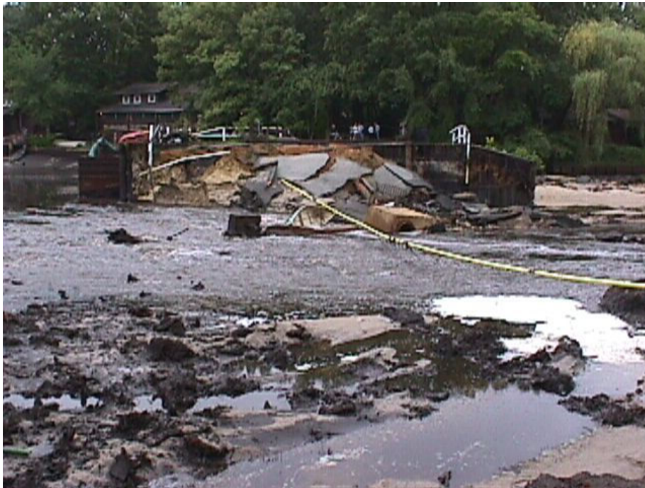
Failure of Upper Aetna Dam in NJ
