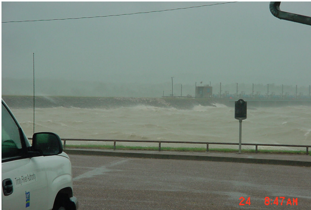
Livingston Dam during Hurricane Rita
